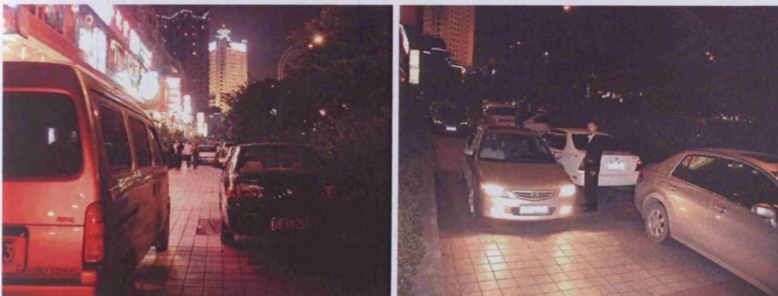
Figure 6.8 Sidewalk deteriorates into a parking space at the busiest time.
