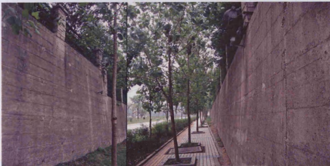
Figure 6.26 The blank concrete wall is used to fence off the sidewalk.
