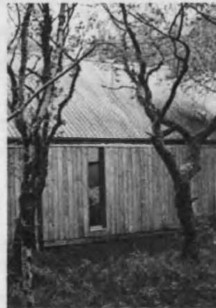
View of the external wall and roof timber boarding
