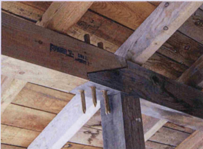
Examples of traditional pegged timber joints
