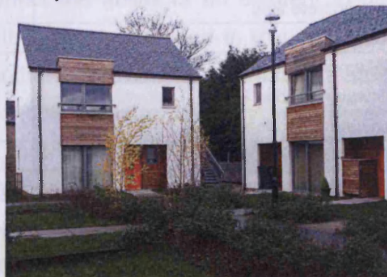
Figure 51 - Toll House Gardens in the Fairfield estate, Perth, Scotland, by Gaia Architects for Fairfield Housing Co-operative
