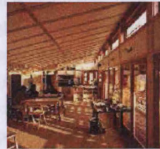
Internal finishing panels divided and fixed through timber trims creating the distinctive Segal aesthetics
