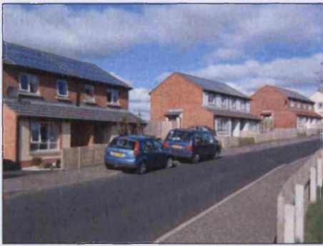
Figure 3-6: Building with building integrated photovoltaic at Derry
