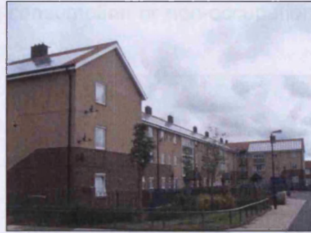
Figure 3-3: Building with building integrated photovoltaic at Newcastle
