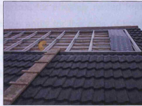
Figure 3-7: The installation of a building integrated photovoltaic system at Nottingham
