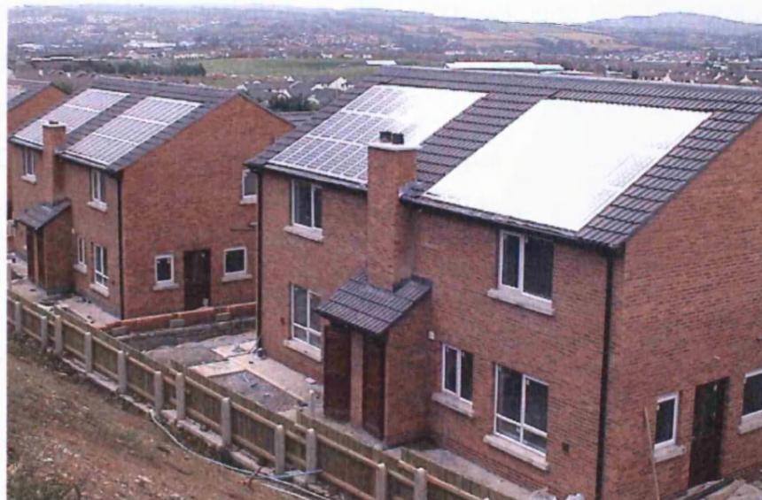
Figure 1-1: Building integrated grid connected photovoltaic system in the urban environment
