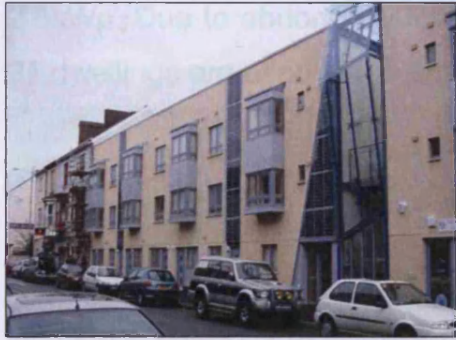
Figure 3-2: Building with building integrated photovoltaic at Llanelli
