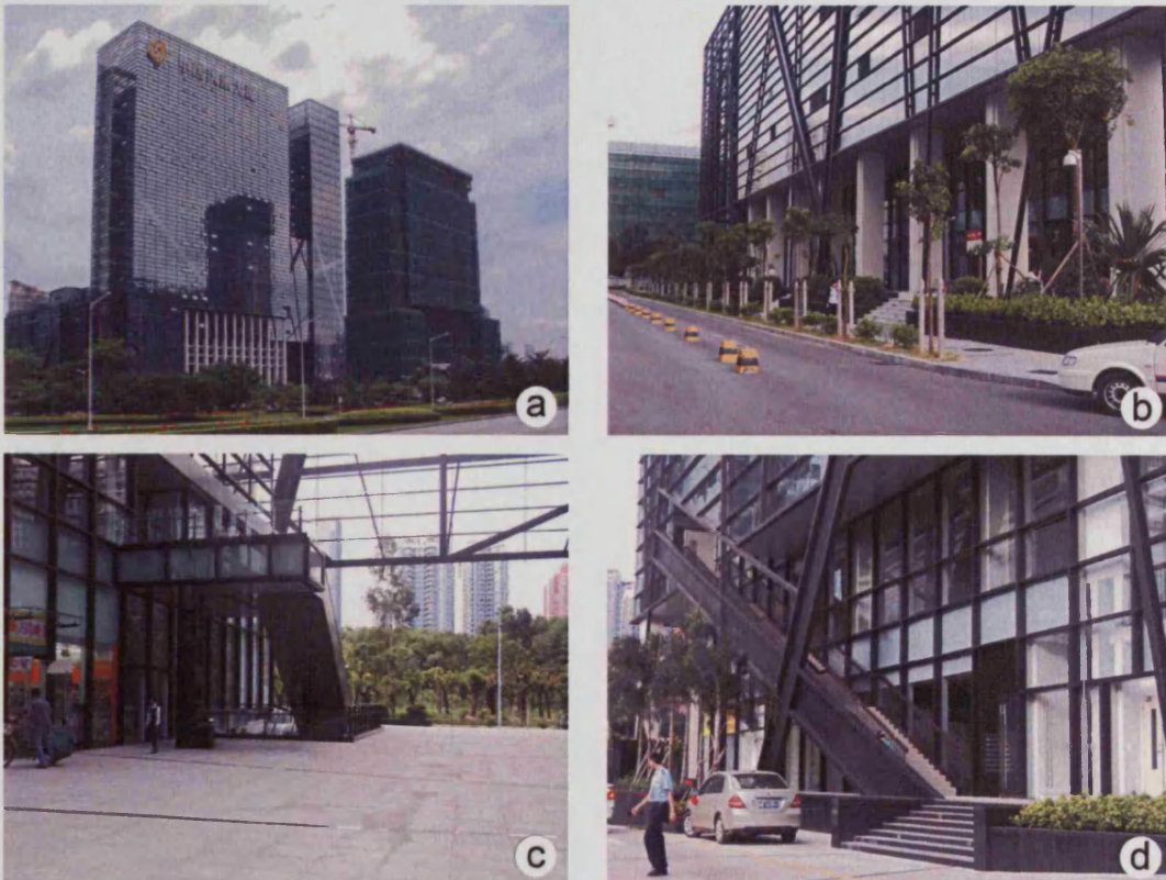
Casefigure 5.8 Phoenix TV Building on site
