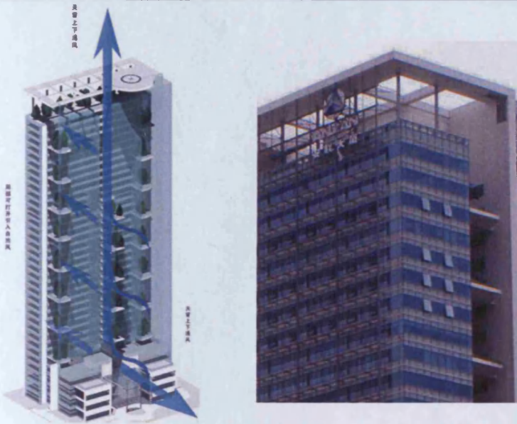
Fig. 7.2.4 The Anlian Tower. The project is marketed as a 'living building' with natural ventilation and multi-level sky gardens (left, by Wong Tung Group) (Source: Huang 2002); sunshade curtains are located on the west elevation to reduce the excessive sunlight, and multi-level sky gardens provide some greenery and joy to the office environment (photo by the author, 2005).
