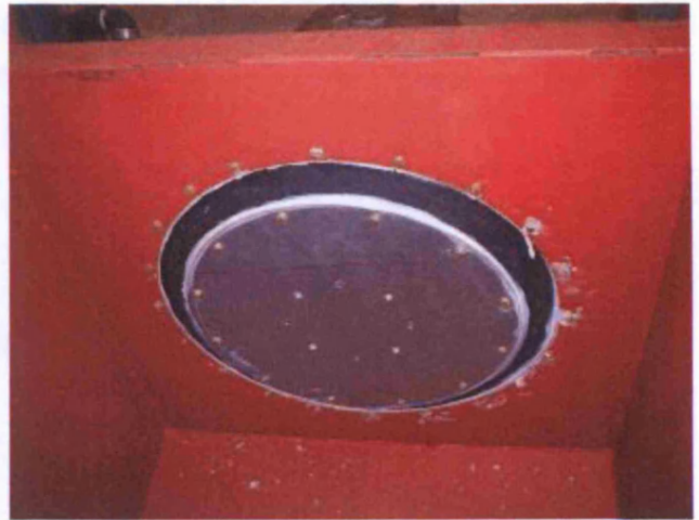
B 3.2 A view of the actuator plate taken from within the bath Note: The plate is not aligned with the inside of the bath because the water has been drained.
