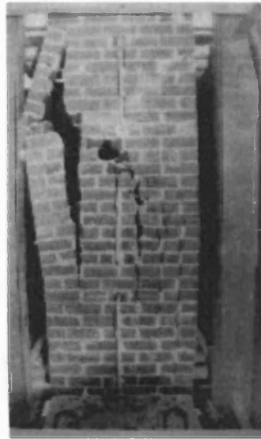
Figure 3-4 – Failure of a brick column
