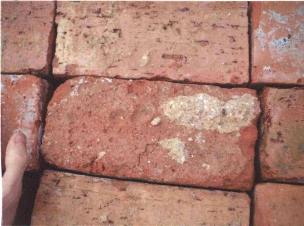
Figure 2-10. Close-up of soft red bricks
