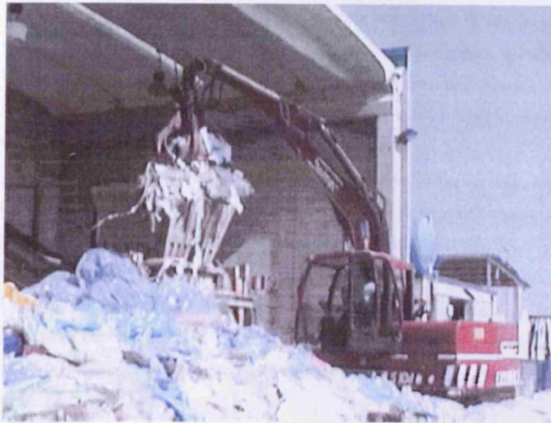
Figure F1 Unsorted plastic film being unloaded from bales.
