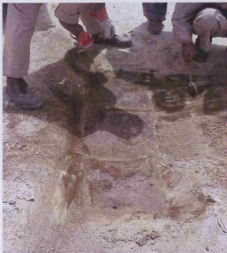
Plate 8.6. Removal of loads and preparation for field testing
