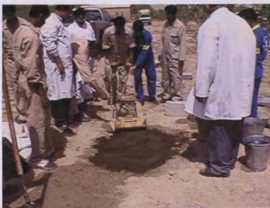
Plate 8.3. Backfilling and compacting the test beds
