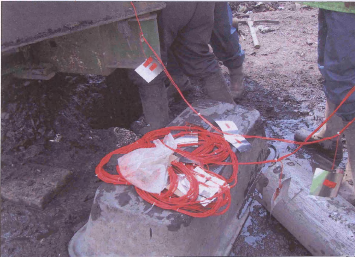
Figure 6.4: A photograph illustrating a pre-fabricated electrode array comprising single-core electrical cables and stainless steel sheet electrodes prior to emplacement within the landfill (Jeremy Jones, Encia Consulting Ltd).
