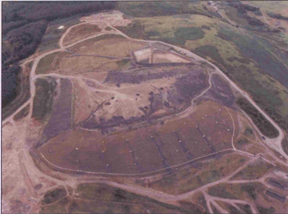
Figure 3.23: An oblique aerial view towards the south taken in 2003 illustrating the Nantygwyddon site after closure (Amgen Rhondda Ltd).
