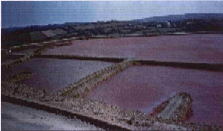
Figure 4.13: Clemows Valley tailings dam, with paddocks
