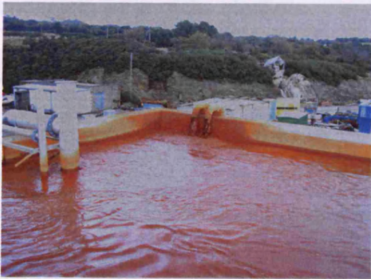
Figure 4.11: Stage I reactor
