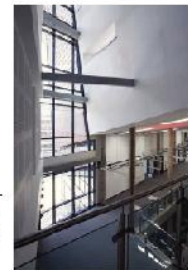
Passive Design utilising exposed concrete ceiling and good daylight design at the Roland Levinsky Building, Plymouth
