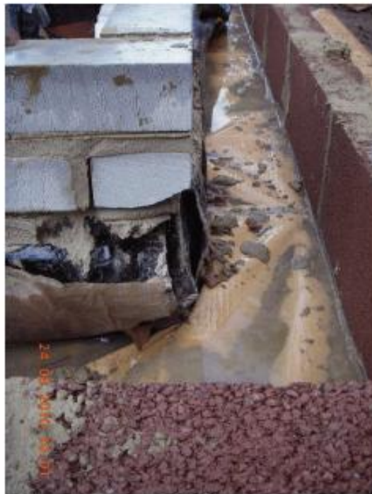
Photograph 5 – Example plot 2 difficulty forming external corner
