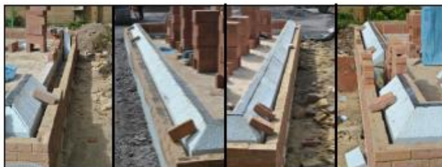
Photograph 6 – Insulation in cavity plot 1 (front, L/H, R/H, rear)
