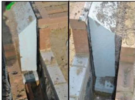
Photograph 6 – Insulation in cavity plot 1 (front, L/H, R/H, rear)
