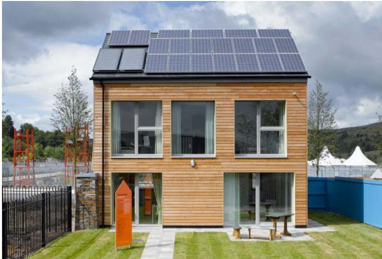
Figure 12 South elevation of the 'Larch' Passivhaus, Ebbw Vale (courtesy of Jefferson Smith)
