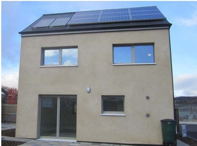
Figure 42 Lime rendered South facade of the Lime Passivhaus, Ebbw Vale
