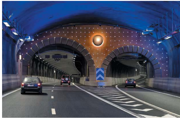
Figure 2.32: The Sodra Lanken Project links east and west of Stockholm's southern side
