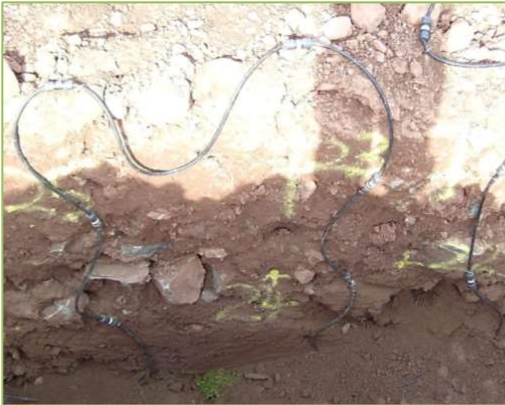
Figure 3.6– Photograph showing part of the installed detailed cross-section BB.
