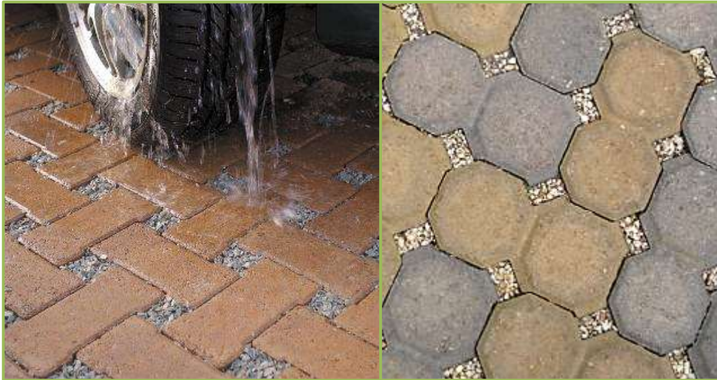
Figure 8.18 – Typical examples of permeable brick paving (Holland Stone, 2013; Quiant Nature, 2013).
