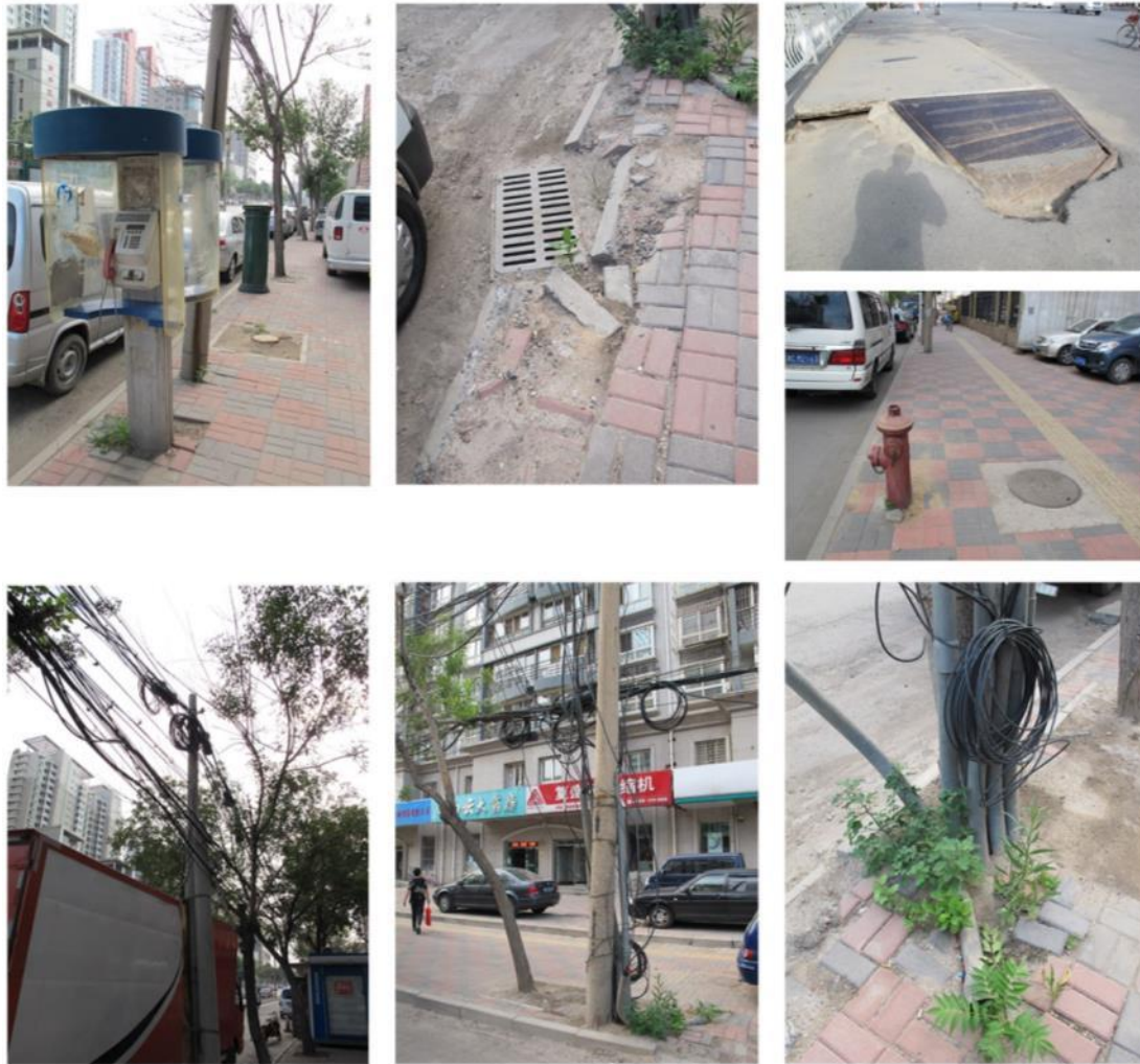
Figure 5-9 Problems of the Infrastructures in the Surrounding Neighbourhood of Case 1
