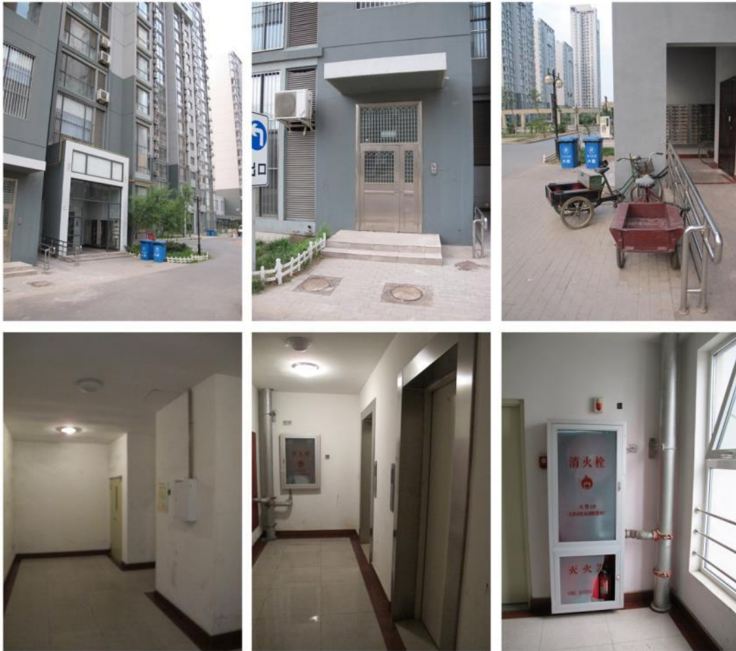
Figure 5- 63 Entrances and Communal Spaces and Facilities of Dwelling Buildings in Case 4
