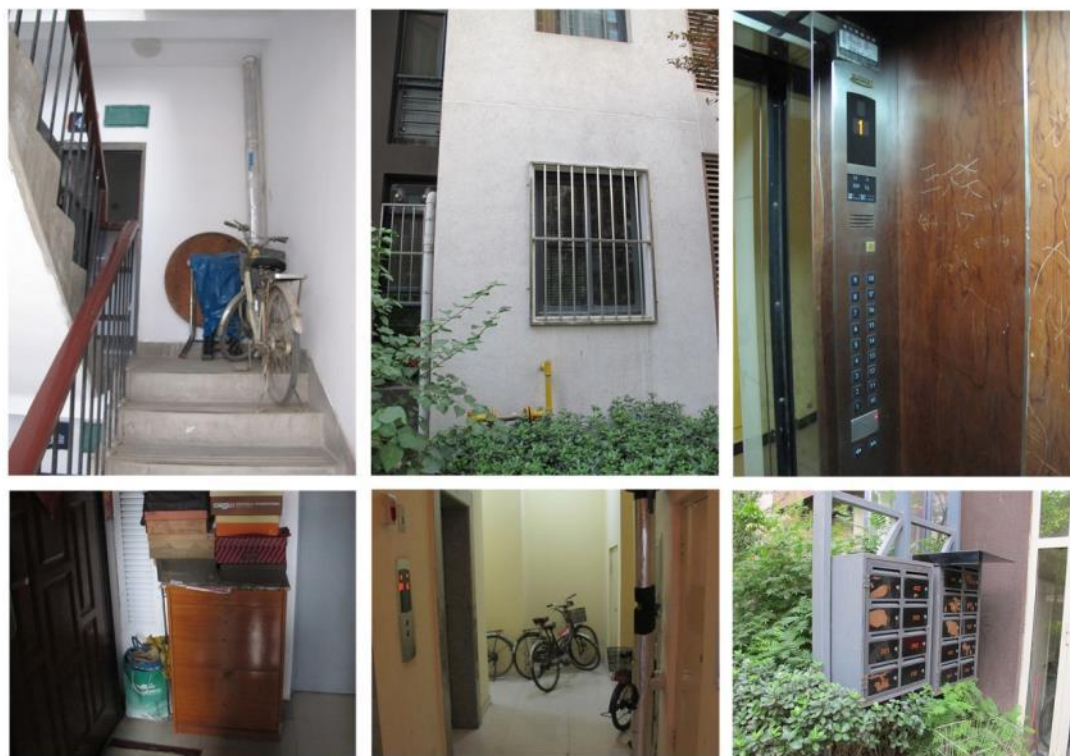
Figure 5-37 Problems of Management and Maintenance of Dwelling Buildings in Case 2
