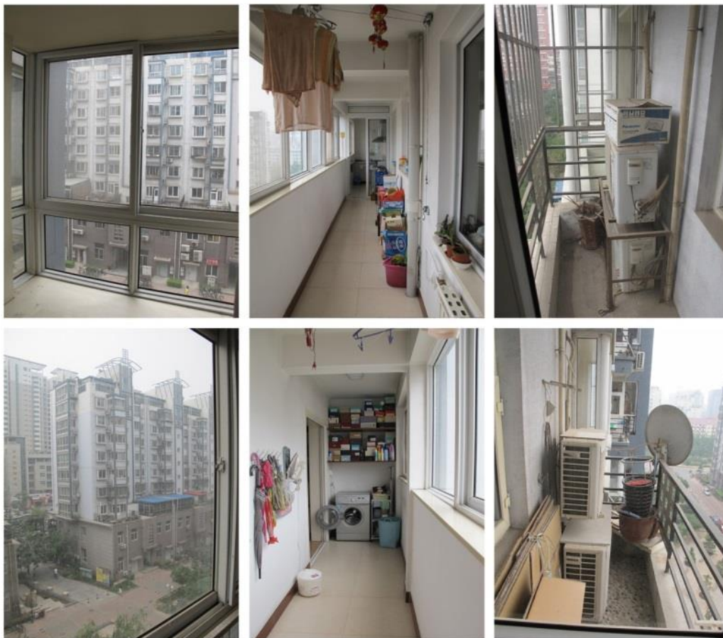
Figure 5- 25 Problems of Dwelling Units in Case 1
