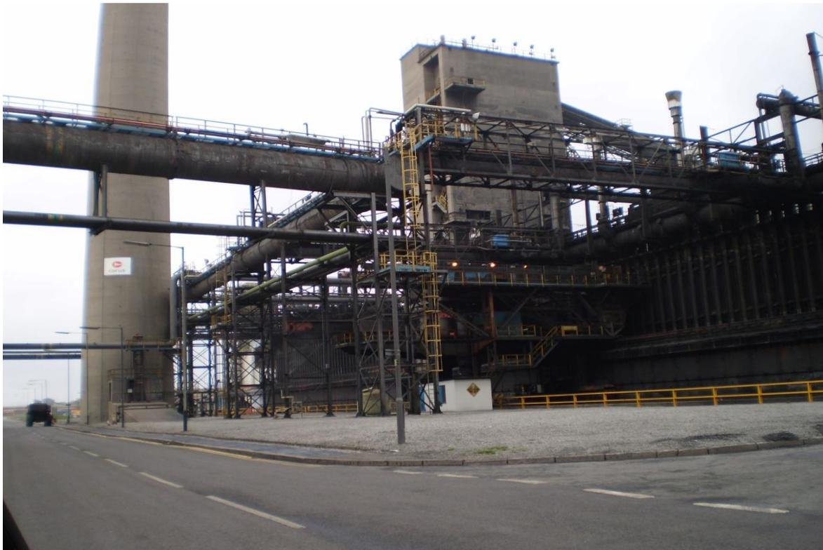
**Figure 4.1** Coke ovens plant at Port Talbot steelworks
