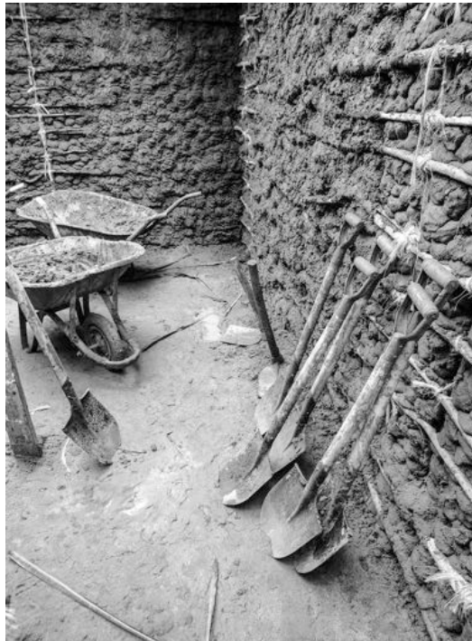
Figure 25. A view inside one of the houses being constructed. Source: Author.
