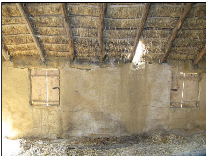
Figure 6.11 Experimental hut at Sarakini (Rhodope, Greece): interior view showing the parallel rafters, side purlins and the thatch cover used for the roof (photo: D. Kloukinas, permission: N. Efstratiou).
