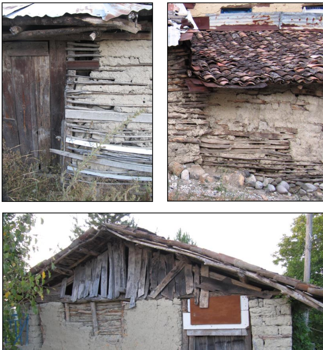
Figure 5.72 The use of planks for the reinforcement or screening of the timber frame at Omorfokklisia (Kastoria, Greece) (photo: D. Kloukinas).
