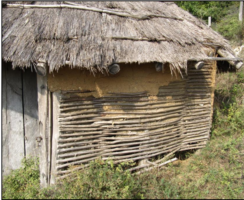
Figure 5.63 Experimental hut at Sarakini (Rhodope, Greece) following the wattle-and-daub technique (photo: D. Kloukinas, permission: N. Efstratiou).
