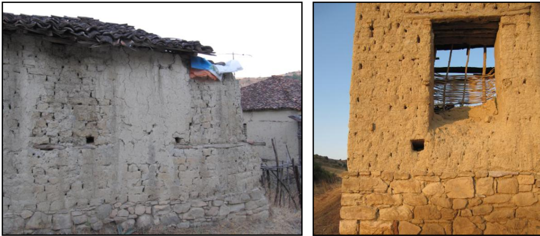
Figure 6.10 Mudbrick buildings with stone foundations from Omorfokklisia (Kastoria, Greece) (photo: D. Kloukinas).
