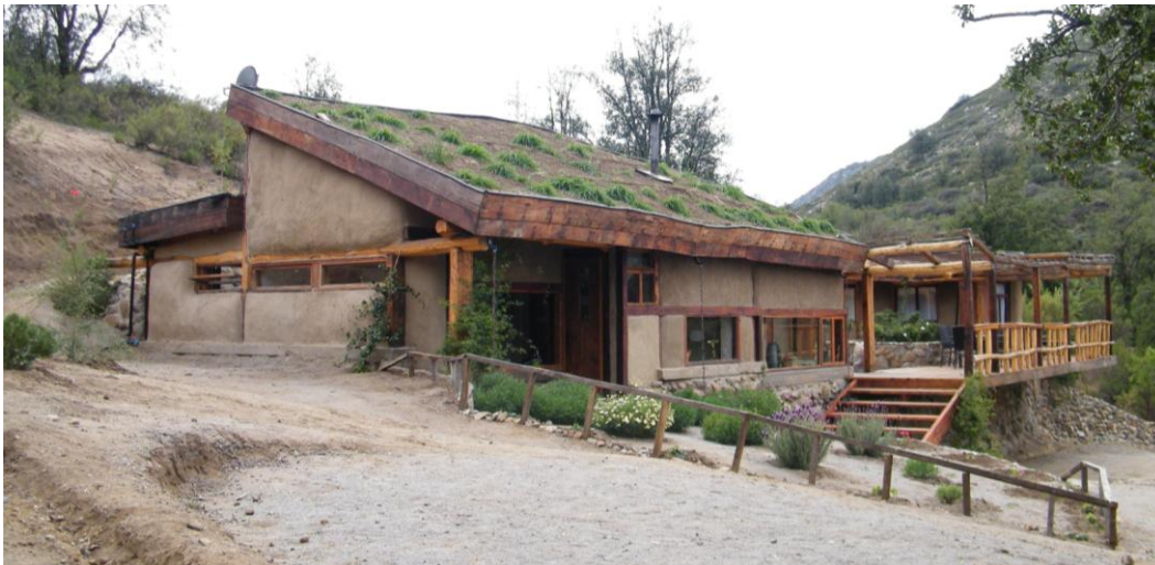
Figure 5. Case Study house Casa Caleu, Caleu, Metropolitan Region, Chile
