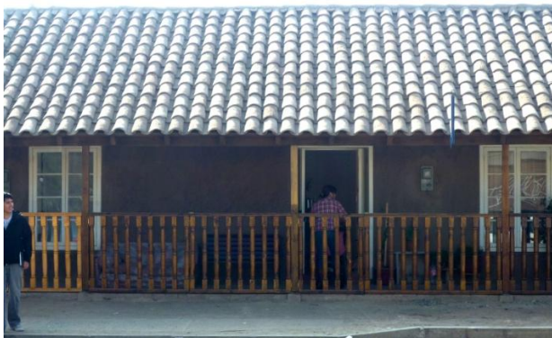
Figure 6: Dwelling rebuilt with straw bales, Chépica, VI Region, Chile.
