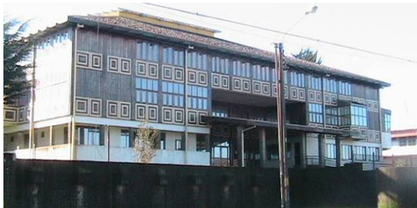
Figure 22. School G, External view
