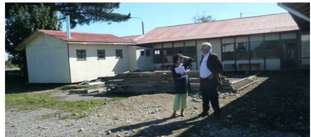
Figure 20. School F, External view
