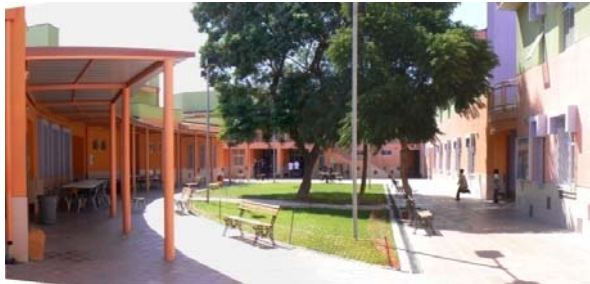
Figure 2. School A, External view
