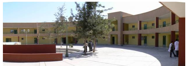
Figure 6. School B, External view
