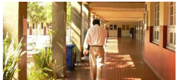
Figure 17. School E, External view
