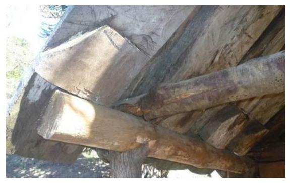
Figure 3. Detail of construction of Pehuenche *fogón*.
