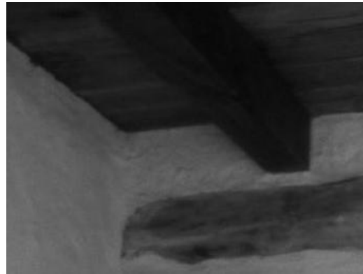
Figure 7: Photograph of wall ceiling-junction.
