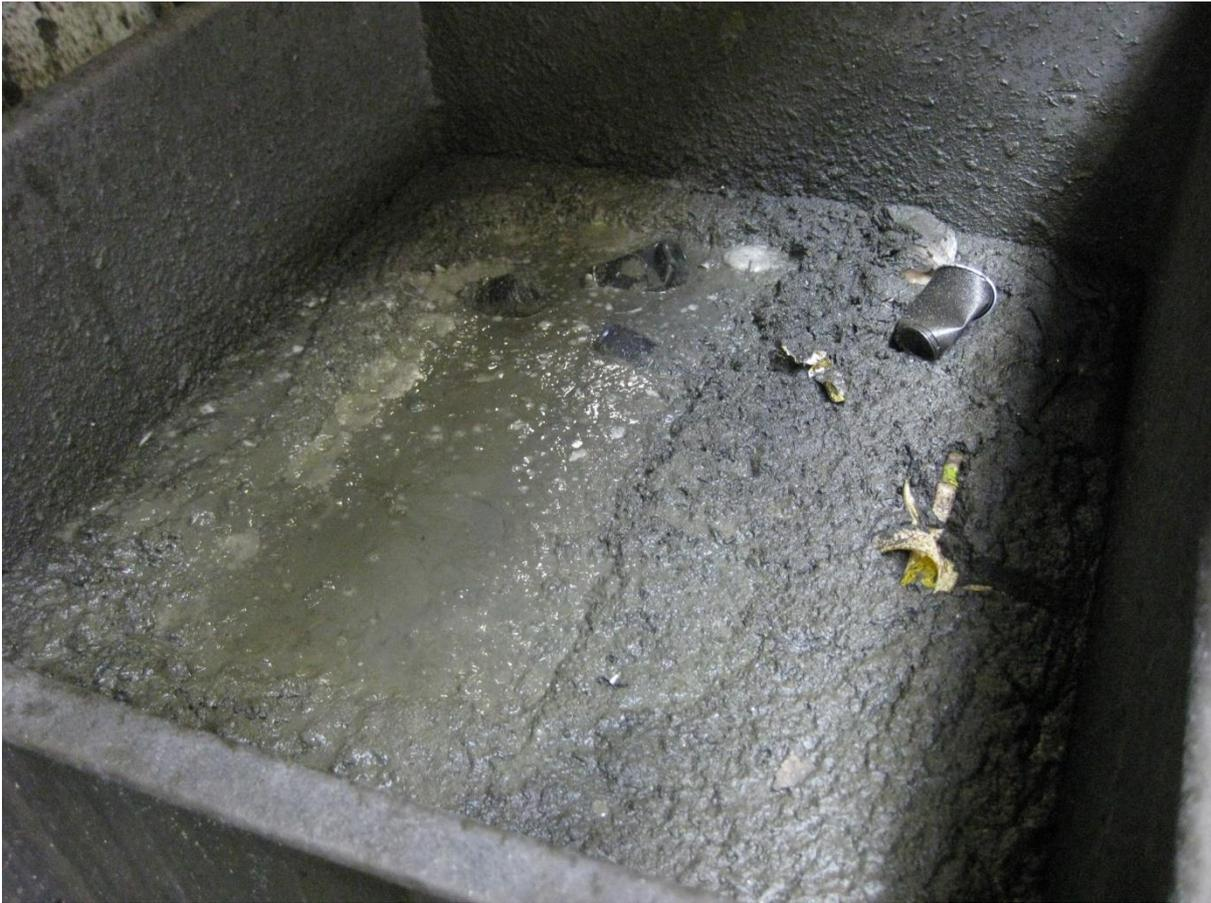
**Figure 14 Sludge Filtered from a Washing System**
