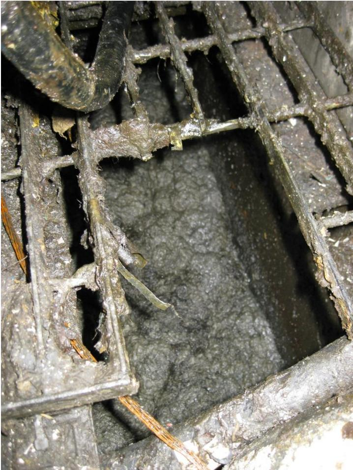
**Figure 13 Sludge within a Sump**
