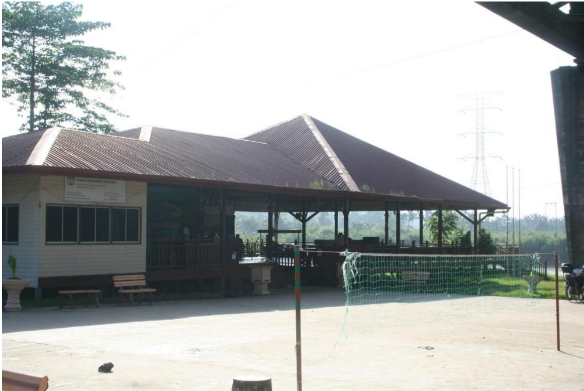
MESCOT Head quarter, which serves multiple purposes of office, reception and community centre
