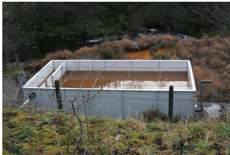
Figure 17: Pilot scale passive system installed by Natural Resources Wales in 2010 for the removal of Zn from the Cwm Rheidol upper adit water.
