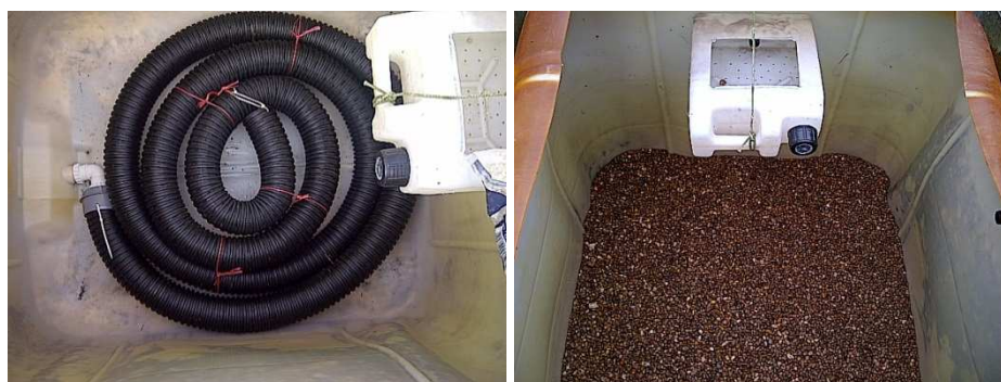
Figure 25: Left is the coiled drainage pipe to the outflow. Right is the gravel layer placed on top of the pipe and the coarse gravel layer.
