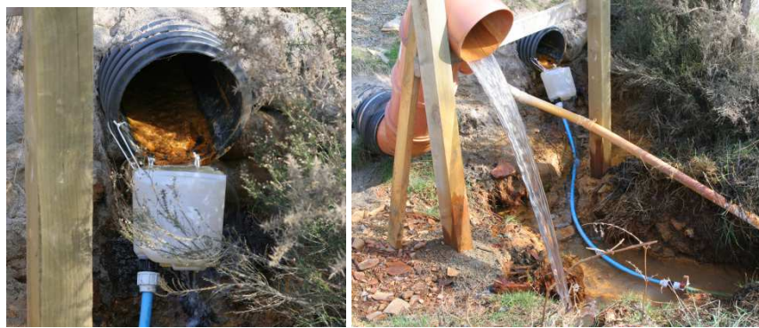
Figure 26: Cwm Rheidol mine water discharge pipes; Left: Is the set up for piping water from the lower number 9 discharge pipe to the VFR. Right: The discharge point of both upper number 6 and lower number 9 adits.
