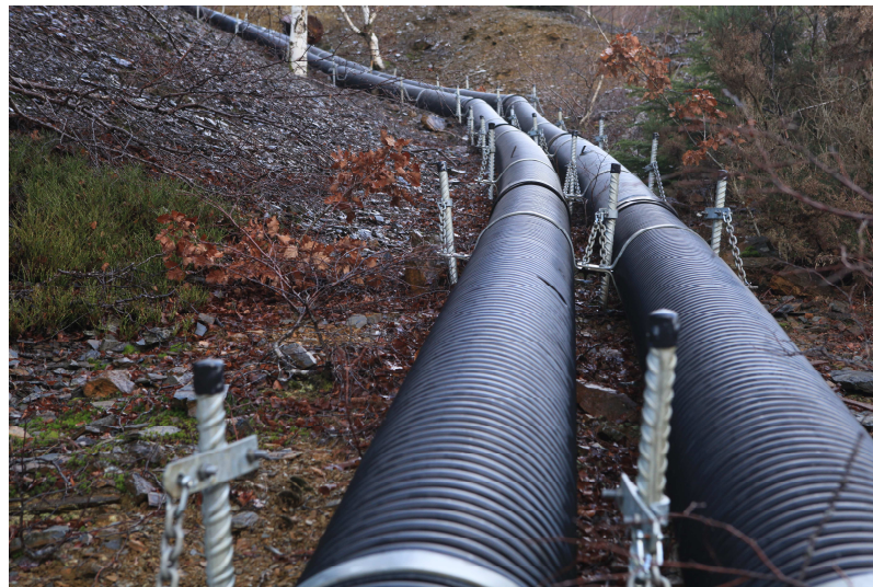
Figure 16: Cwm Rheidol Mine water discharge pipes (left: No. 6 adit, right: No. 9 adit).
