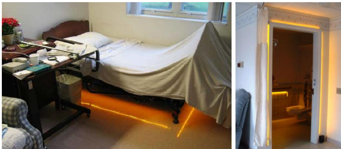
Figure 4.10: Trial observation rooms using amber LEDs around the bed and bathroom doorways (Figueiro & Rea, 2005)
