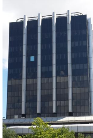
Figure 6.6: Photograph of the external facade of a building with a large percentage of body-tinted glazing (authors own)
