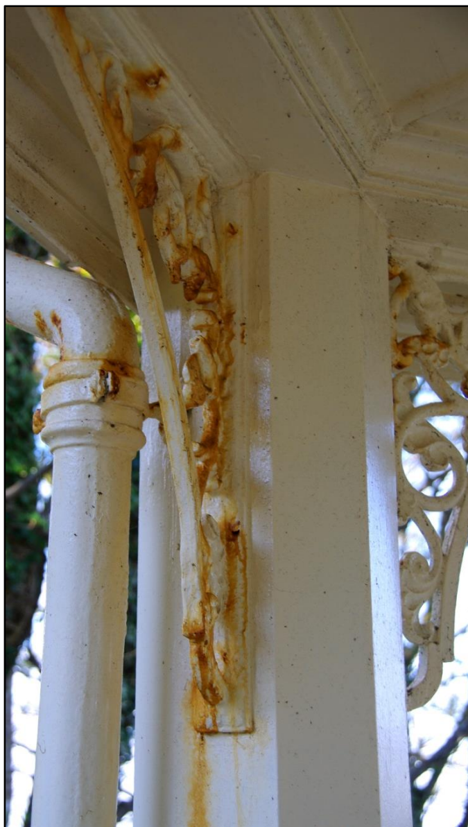
Figure 6.11 Failure of system similar to System A within 12 months of reinstatement in coastal environment. Corrosion staining evident on pale coloured topcoat.
