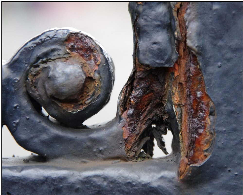
Figure 2.5 Wrought iron gates at the Palace of Holyroodhouse showing coating failure and laminating corrosion of underlying substrate.
