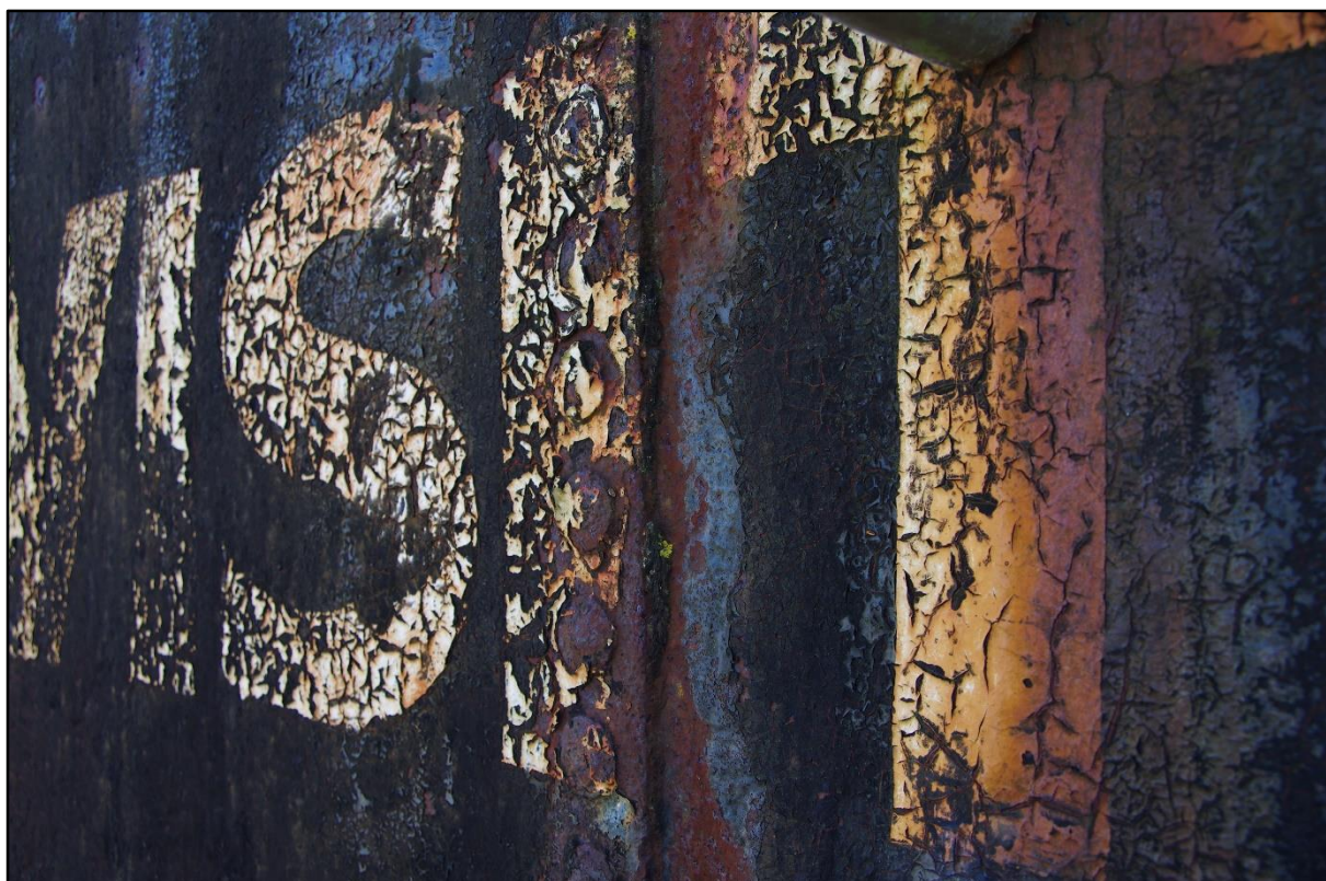
Figure 3.1 Bituminous coating on a brine tank in Cheshire.
