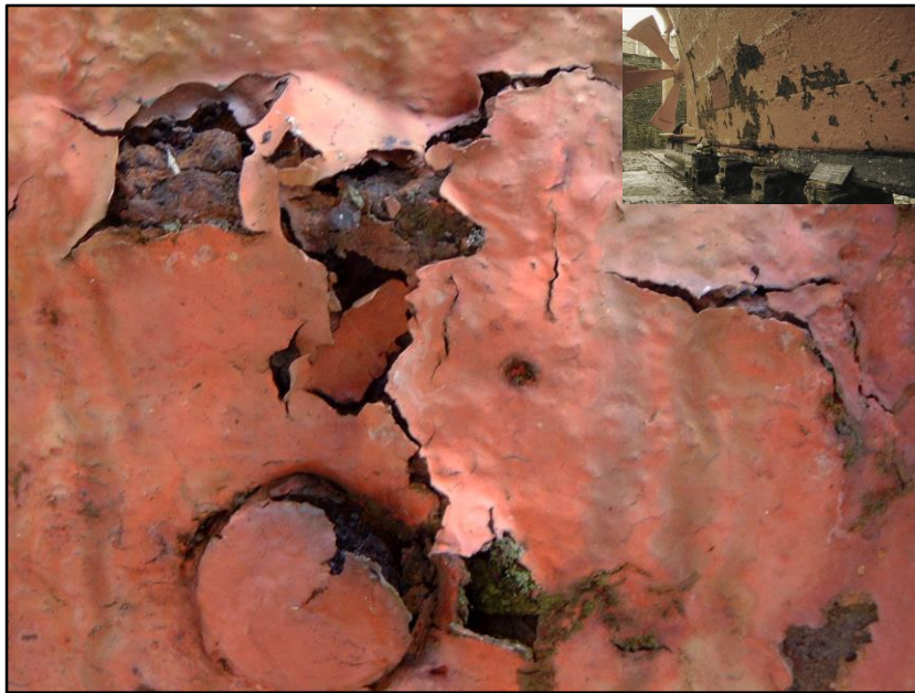
Figure 2.14 Brunel's ss Great Britain paint loss and lamellar corrosion.
