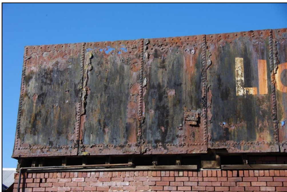
Figure 2.11 Wrought iron brine tank at Lion Salt works Cheshire.
