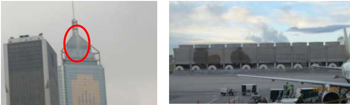
Figure 36 Visible plume discharged from a cooling tower in tall building and airport
