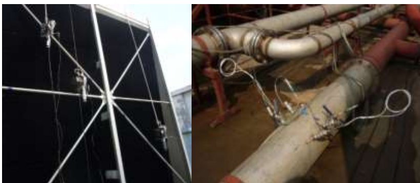
Figure 26 Dry-bulb and wet-bulb temperature sensor at where air is drawn into the cooling tower (Left) Sensors for water temperature at the main pipe (Right)
