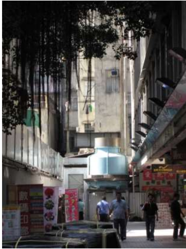
Figure 81 Cooling Tower located close to pedestrian levels
