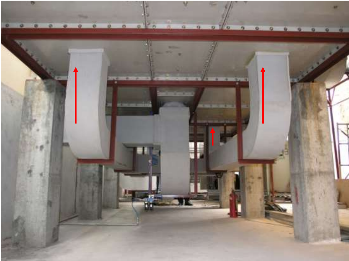
Figure 41 Vent that transports treated air into the testing chamber
