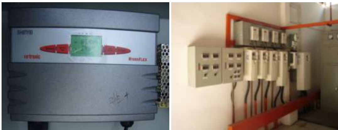
Figure 29 Rotronic HygroFlex - Temperature & RH monitoring equipment (Left) monitoring equipment of the boiler (Right)
