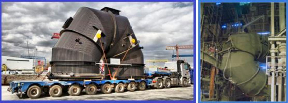
Figure 118 Top Bend of the off-gas system.
