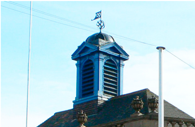
Figure 2. Roof Ventilator: Cradely Heath Library Wills and Anderson, 1909.
