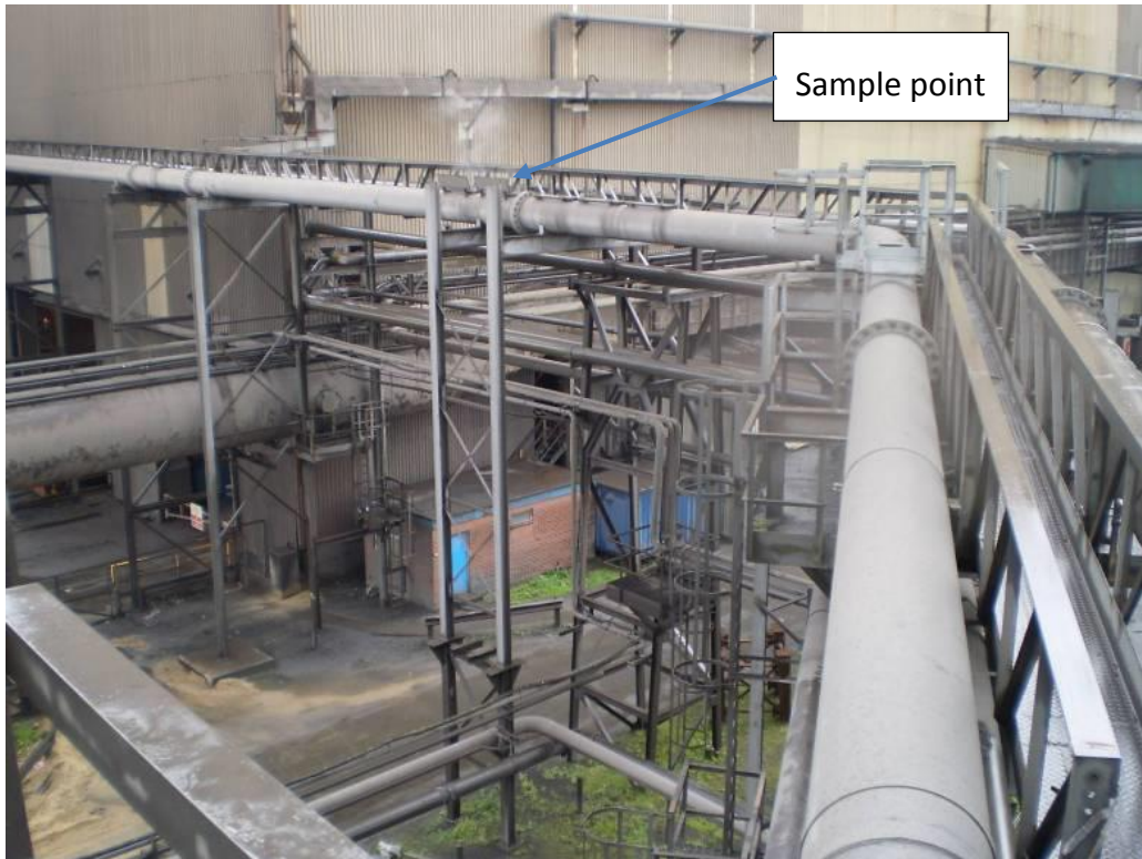
Figure 2. Picture of BOS slurry pipe and sampling point
