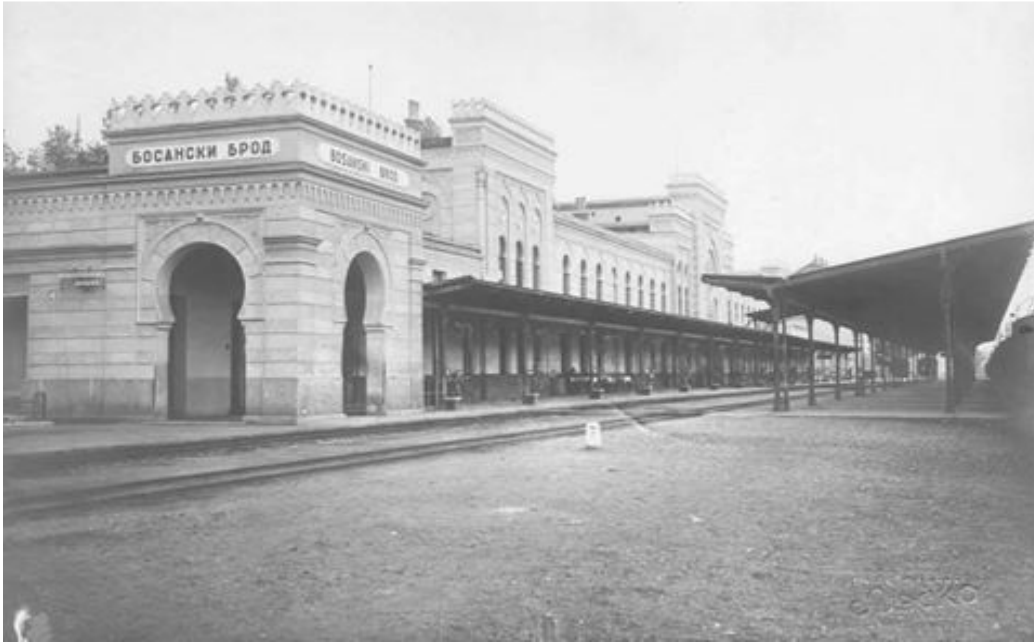
Fig. 5.7 – The Railway Station at Bosanski Brod, erected in 1896, after the design of an Austrian architect Hans Niemeckz. Destroyed in 1945, now in ruins.
