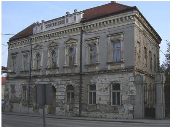
Fig. 2.58 – Damage to the Serbian Home in Vukovar, erected in 1905 in place of the 1733 Serbian-Russian-Church-Slavonic School .
