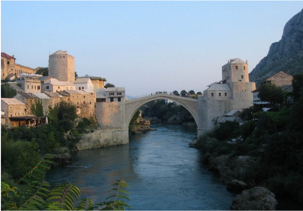
Fig. 5.15 – The Mostar Bridge, built by an apprentice of Mimar Sinan in 1566 on place of an older Mediaeval bridge, destroyed in 1993 by Croat forces in Herzegovina. Rebuilt in 2004 by various international agencies, without participation of local conservation experts. Inscribed in the UNESCO's World Heritage List in 2005.
