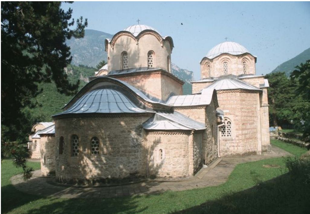
Fig. 3.28 – The Patriarchate of Peć, Monastery church, erected in 1346 in the Raška Style of architecture .
