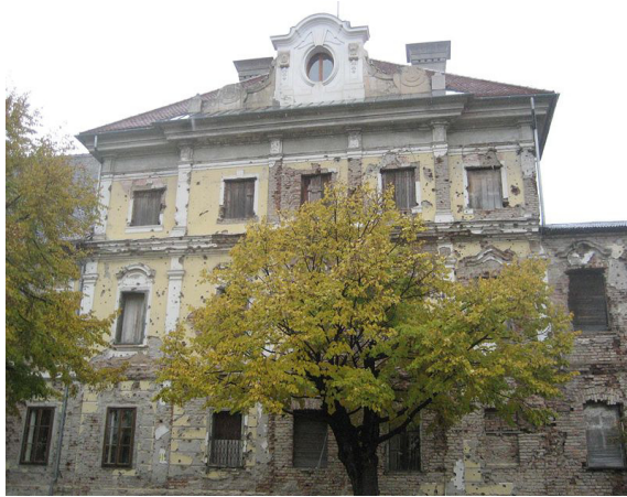
Fig. 2.57 – Damage to the Eltz Manor in Vukovar in 1991. Built in 1749-1751 for the German noble, Karl von Eltz-Kempenic.
