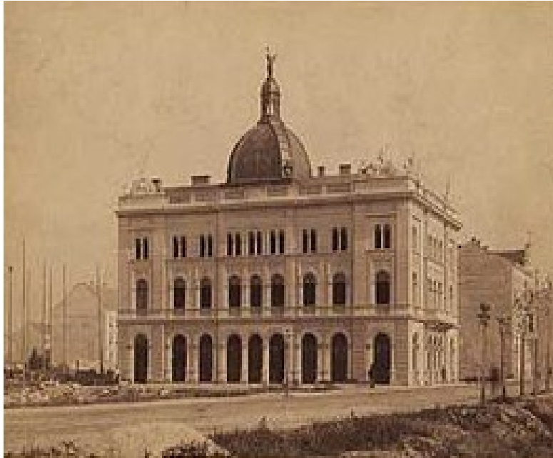
Fig. 2.31 – Starčević’s town house, erected on the newly built Starčević’s Square in Zagreb. Funded by donations of his followers, the house was designed by German architects Leo Hönigsberg and Julio Deutsch in Italian Neo-Renaissance style. The archival photograph was taken by the first Zagreb photographer immediately after the completion.
