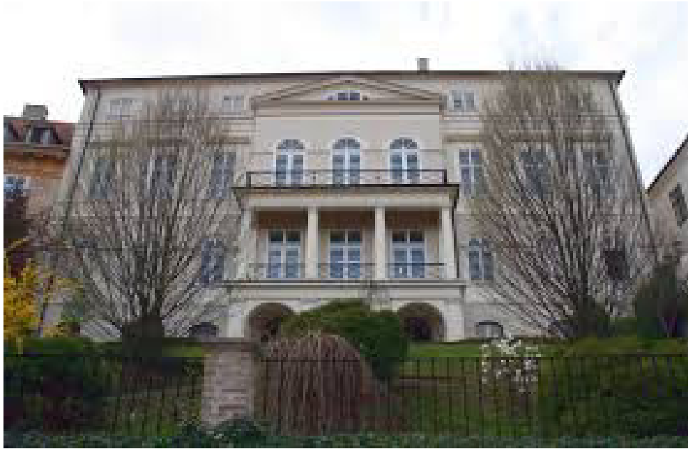
Fig. 2.8 – The Drašković town palace where the National Museum was first housed. Designed and erected in the Neo-Classical style in 1838 by the Czech architect Bartol Falbinger (1785-1871). Today it serves as a municipal building Narodni dom (National Home) and houses the Institute for Croat Language, Theatre and Music.
