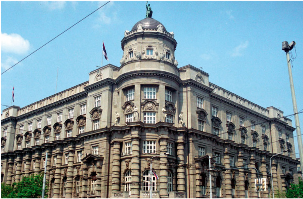
Fig. 1.44 – The building of the Ministry of Foreign Affairs and Ministry of Finances, designed and erected in neo-Classical style by Nikolai Krasnov in 1928-1938.
