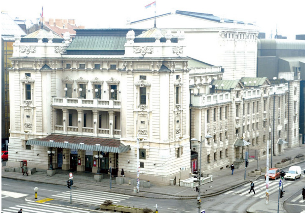
Fig. 1.12 – The National Theatre, modern façade. After the destruction in the First World War, it was rebuilt on a more modest scale. Damaged again in 1941.
