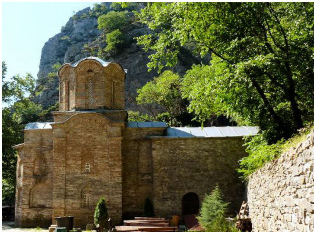
Fig. 4.38 – St. Andrew's Monastery in Treska Canyon
