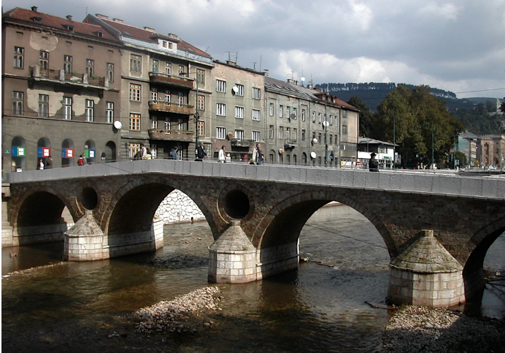
Fig. 5.26 – Erected in the late 18 th century by the Ottomans, after the Austro-Hungarian occupation in 1878, the bridge was repaired and named the Latin Bridge . It gained fame as a place of the assassination of Arch-duke Franz Ferdinand on 28 June 1914. The date of the Austro-Hungarian military manoeuvres was deliberately chosen to coincide with the Serbian national day, Vidovdan , the date of the eponymous Kosovo Battle . During both Yugoslav eras, the bridge was renamed into the Princip's Bridge , in honour of Gavrilo Princip, only to have the name Latin Bridge restored after the Yugoslav wars of succession.
