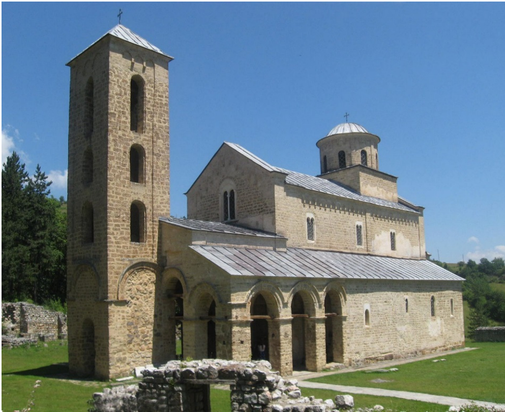
Fig. 1.61 – The Sopoćani Monastery, built around 1260s, is the first example of the Raška School to be listed by UNESCO as World Heritage Site in 1979.
