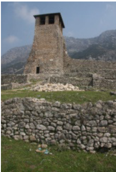
Fig. 3.10 – The remaining original watchtower at Kruje.
