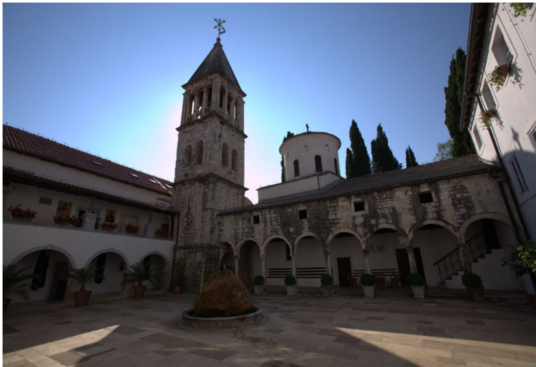
Fig. 2.69 – The Monastery of Krka, erected in 1345 on the old Roman ruins as endowment of Princess Jelena Nemanjić-Šubić. Built partly in the Romanesque style, with later additions. Survived the Second World War and partly demolished in the 1990s. Renewed in 2001.
