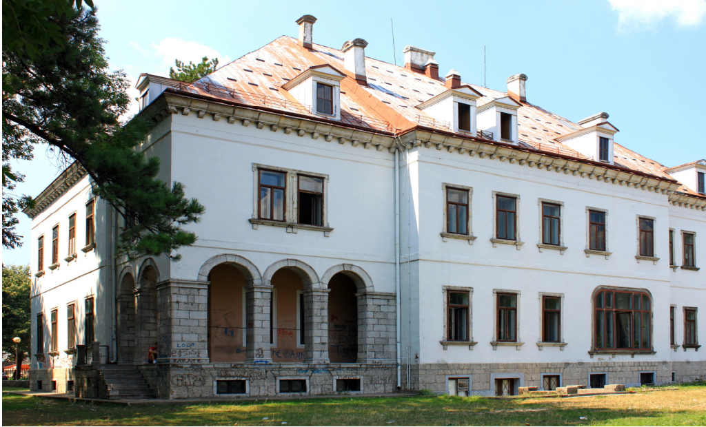
Fig. 6.23 – Building of the former Austro-Hungarian Embassy, built in 1897-1899 after the designs of Josip Slade, now the Institute for Protection of Monuments of Montenegro.
