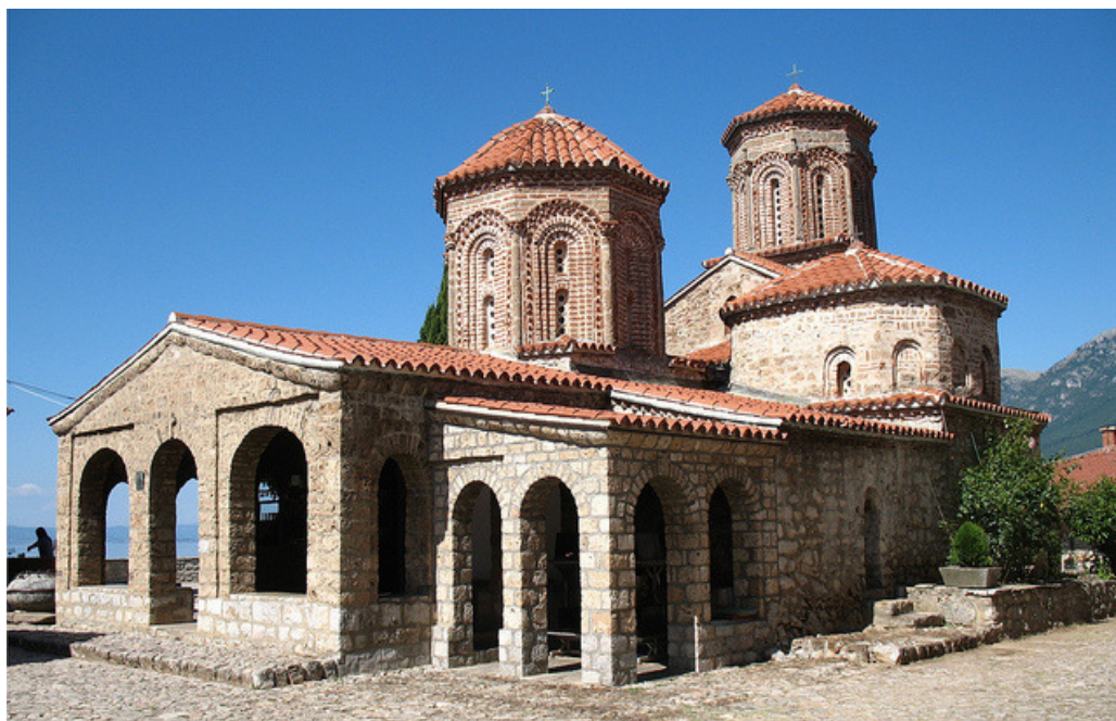
Fig. 4.32 – The Monastery of St. Naum, Ohrid, late 9 th century. Byzantine style of architecture re-named into Macedonian school of architecture
