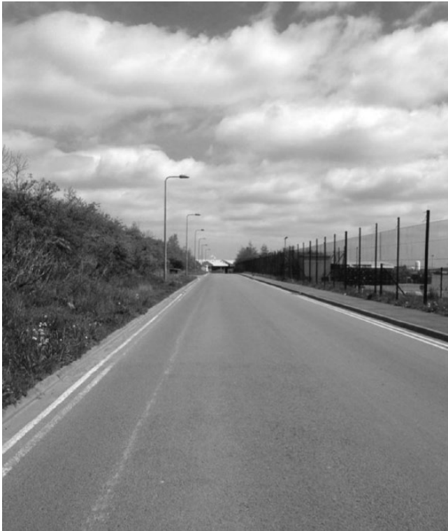
Figures 1 and 2. The Road to Nowhere: The approach to a meat-processing factory near Merthyr Tydfil in the Welsh Valleys.
