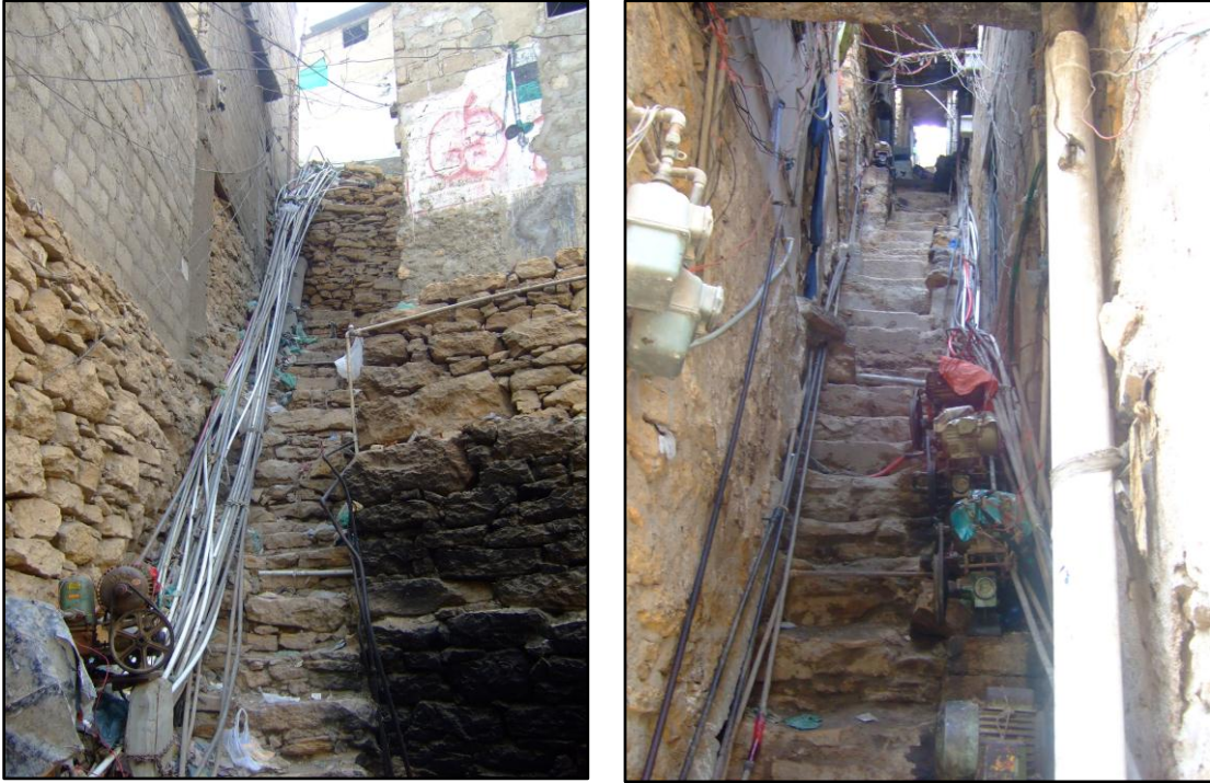
Picture 6.6: Stepped streets, leading to the hill, lined with water pumping equipment and the lines in Chamra Chum area
