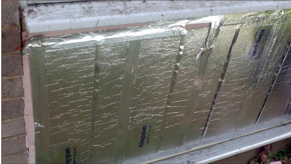
Figure 39: Photograph showing vacuum insulation panel installation, showing failure of foil tape vapour occlusion
