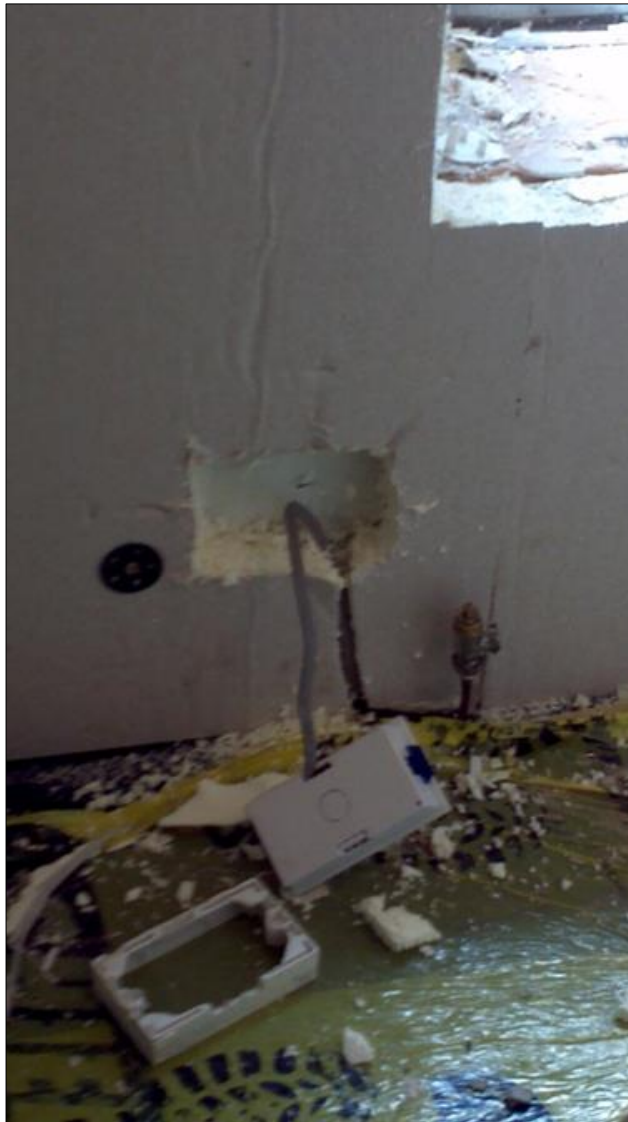
Figure 33: Photograph showing electrical fitting relocated in IWI installation
