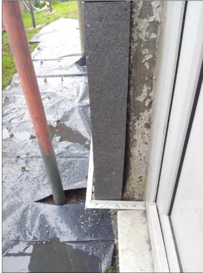
Figure 45: Photograph showing gap behind insulation board due to a 'bell' in existing wall
