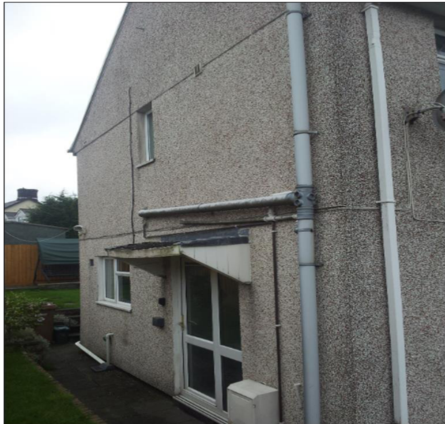
Figure 54: Photograph showing multiple service mountings and penetrations, as well as projecting porch roof prior to EWI installation.
