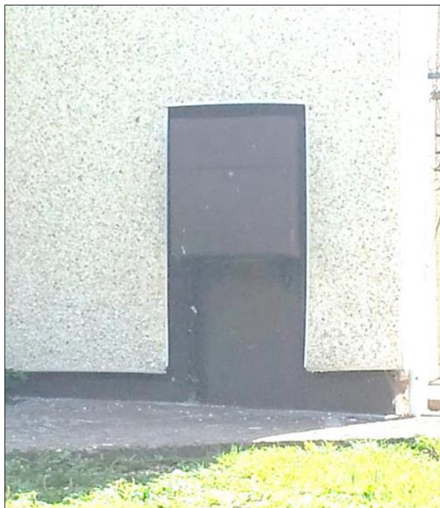
Figure 22: Photograph showing uneven edges around gas meter box
