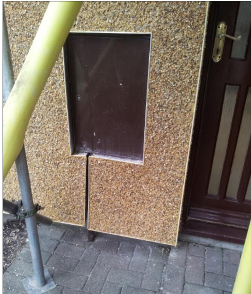
Figure 44: Photograph showing gas supply line and shut-off valve blocked by EWI
