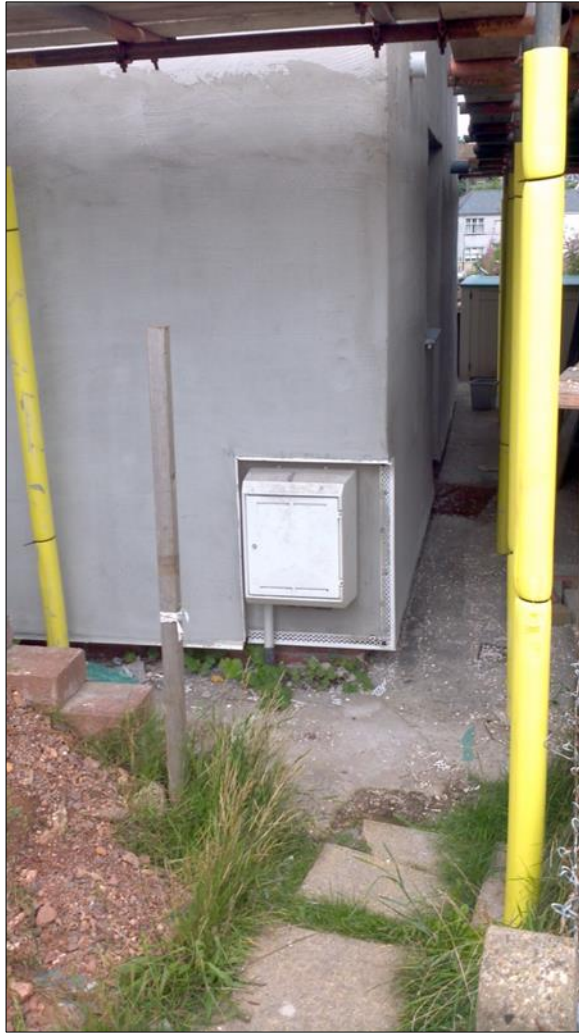
Figure 50: Photograph showing uninsulated area around gas meter
