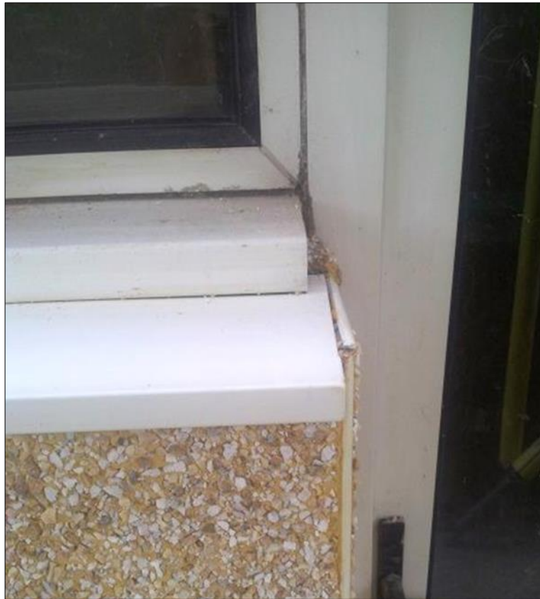
Figure 31: Photograph showing insulation board extended beyond cill and undercill
