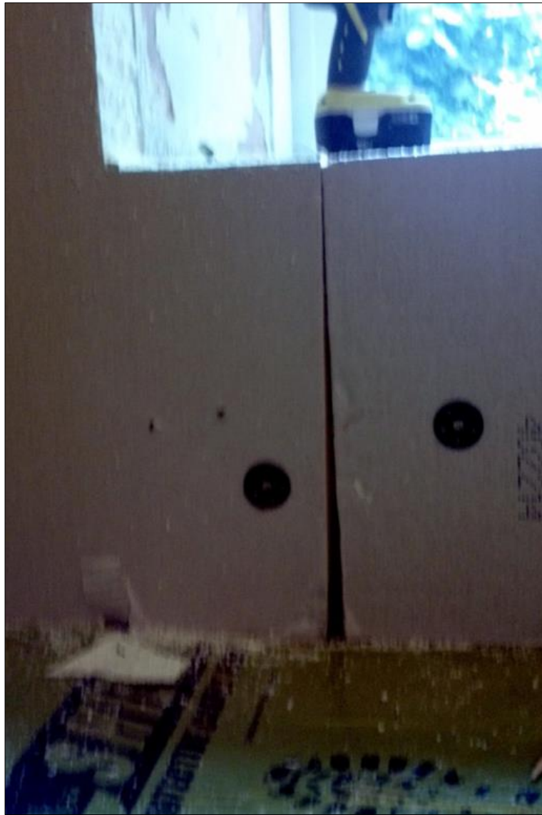
Figure 32: Photograph showing large gap between IWI boards and incorrect locations of pins
