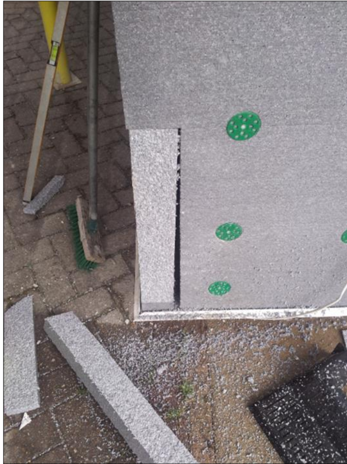
Figure 46: Photograph showing gap behind insulation board due to a 'bell' in existing wall and poor butting of adjacent board
