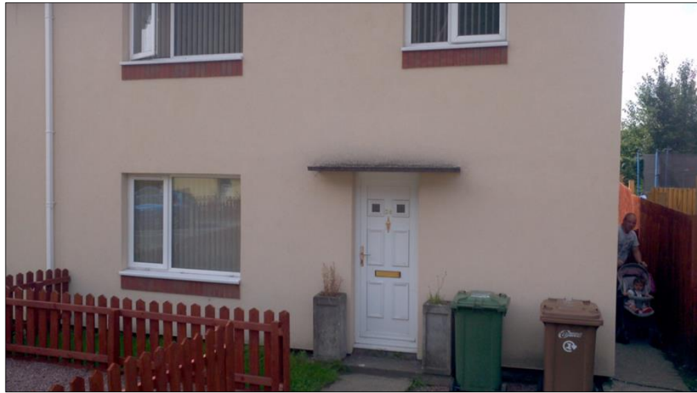
Figure 56: Photograph showing soiled area on EWI caused by splashing from porch roof
