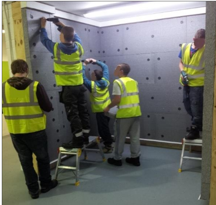
Figure 73: Photograph showing NVQ 2 apprentices practicing 'domino' pinning in Training School 2
