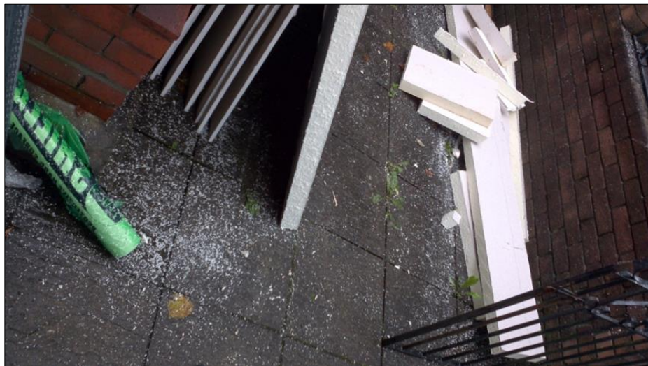
Figure 24: Photograph showing polystyrene waste from cutting of EPS
