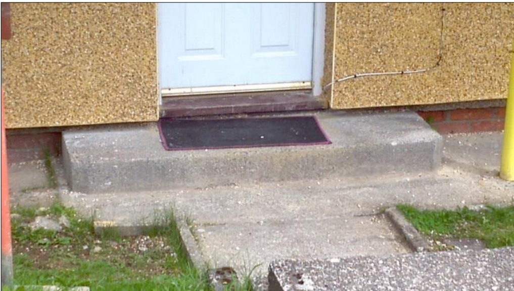
Figure 29: Photograph showing additional example of appropriate practice offsetting EWI over doorstep to protect from moisture
