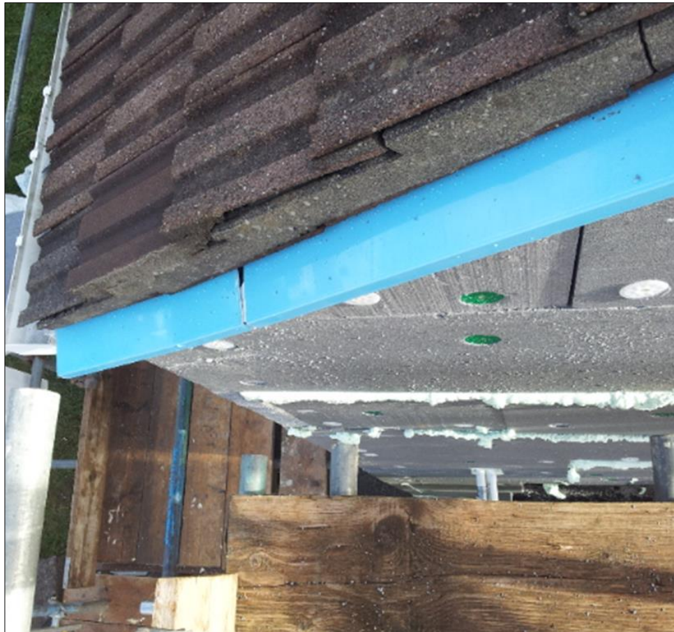
Figure 27: Photograph showing gap between verge trim segments
