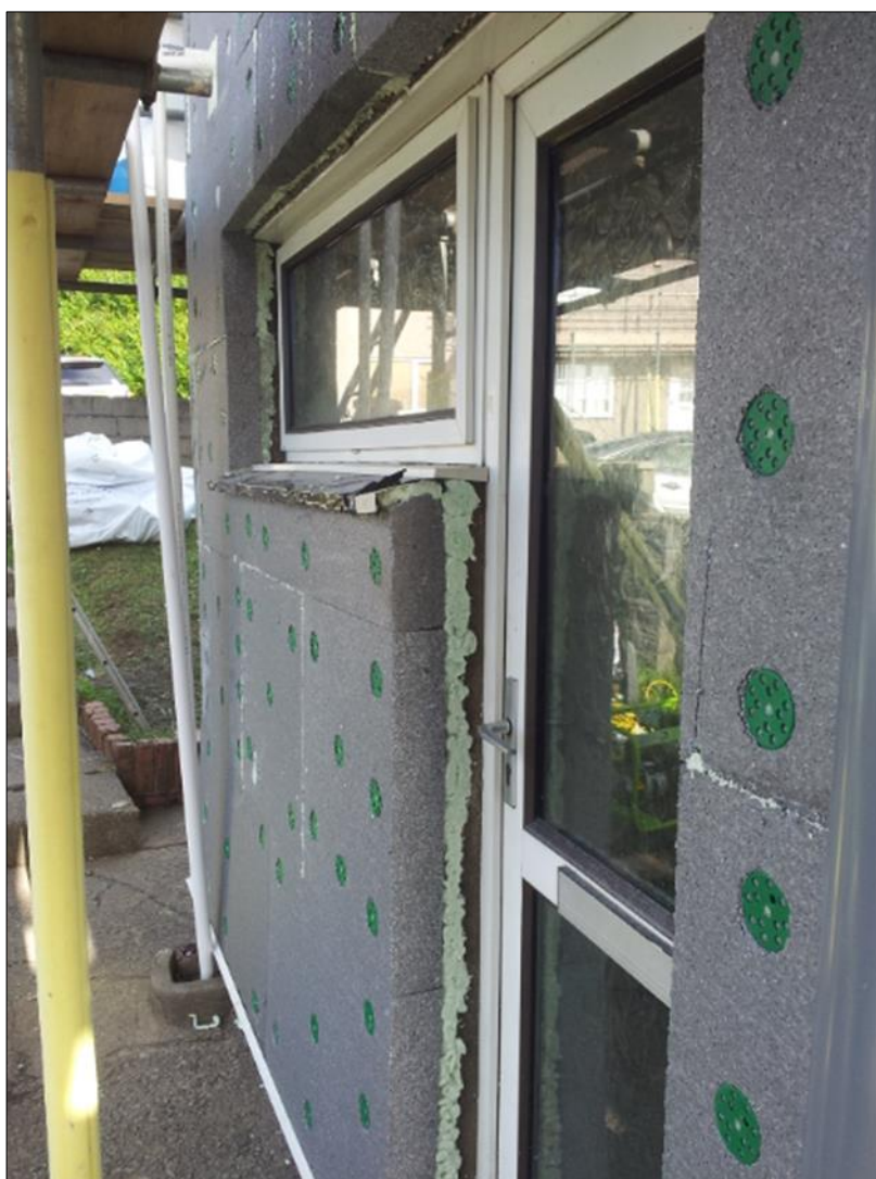
Figure 47: Photograph showing gap behind EWI insulation board
