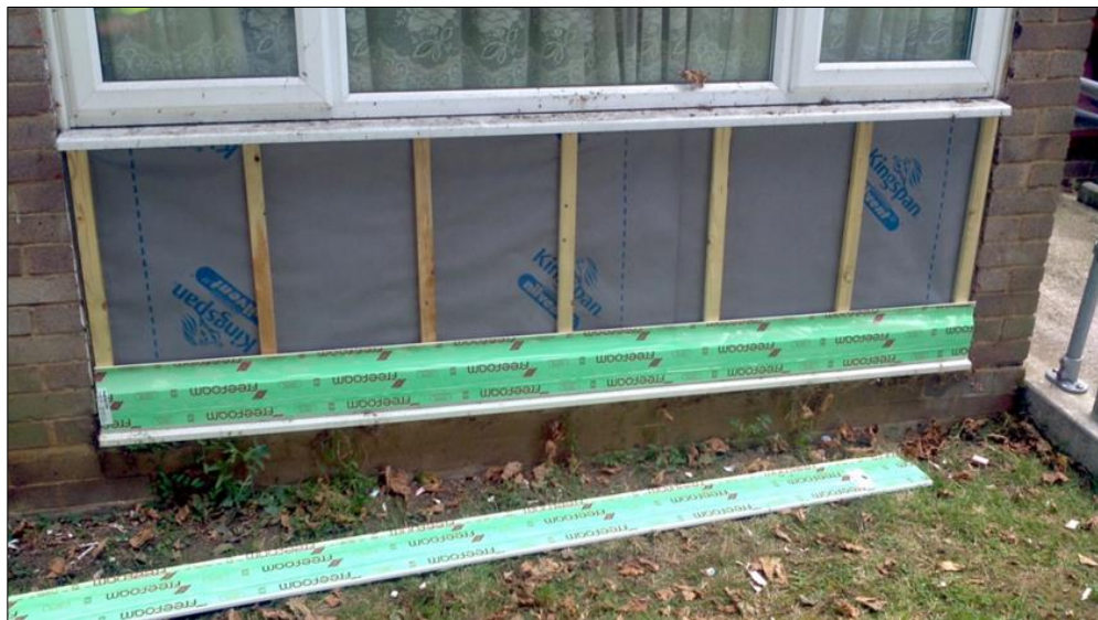
Figure 38: Photograph showing vacuum insulation panel installation, showing difficulty of vapour occlusion
