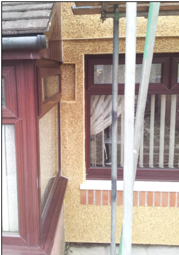
Figure 59: Photograph showing EWI cut away to accommodate outward-opening window
