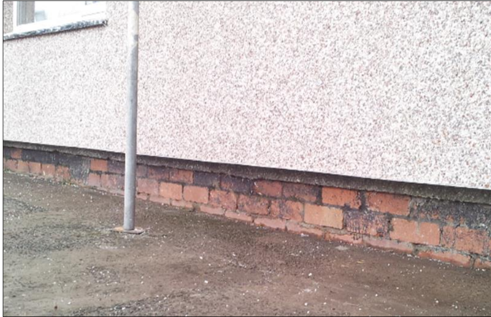
Figure 48: Photograph showing uninsulated wall-floor junction
