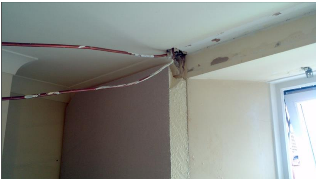
Figure 35: Photograph showing practice typical of observed IWI installations. Note large uninsulated area at ceiling-floor void and open pathway for vapour movement around pipes
