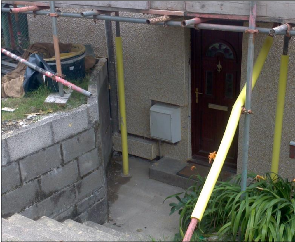
Figure 51: Photograph showing uninsulated wall area around gas meter, gas supply, and soil pipe.
