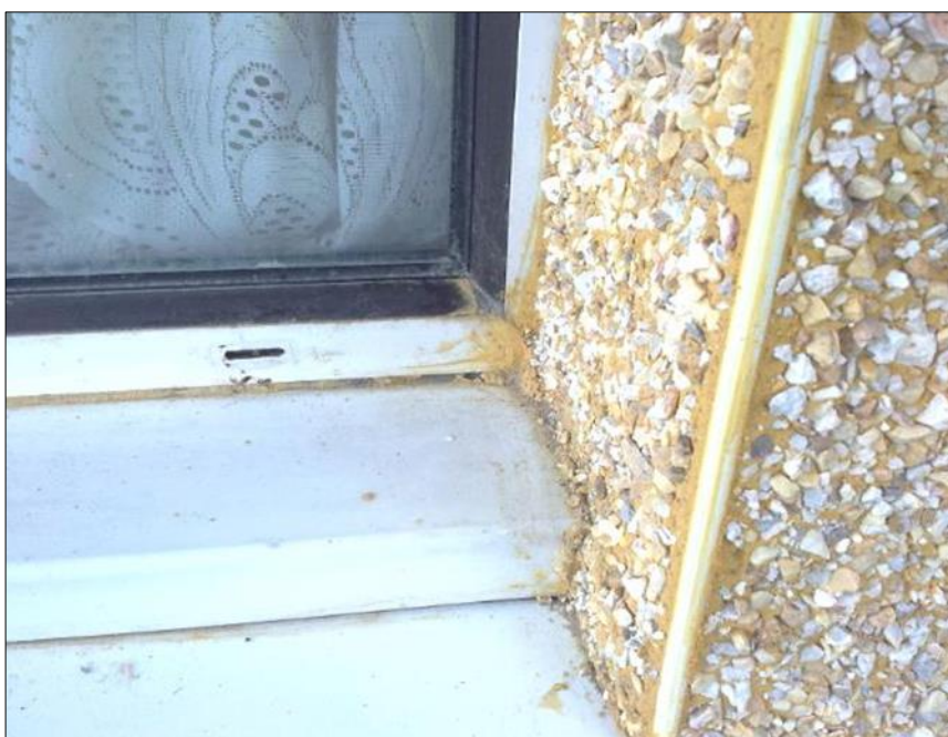
Figure 21: Photograph showing render on window, cill and cornerbead
