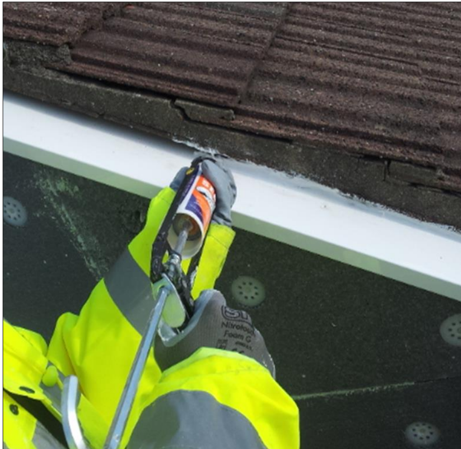
Figure 26: Photograph showing a large gap between verge trim and roof sealed with silicone caulking
