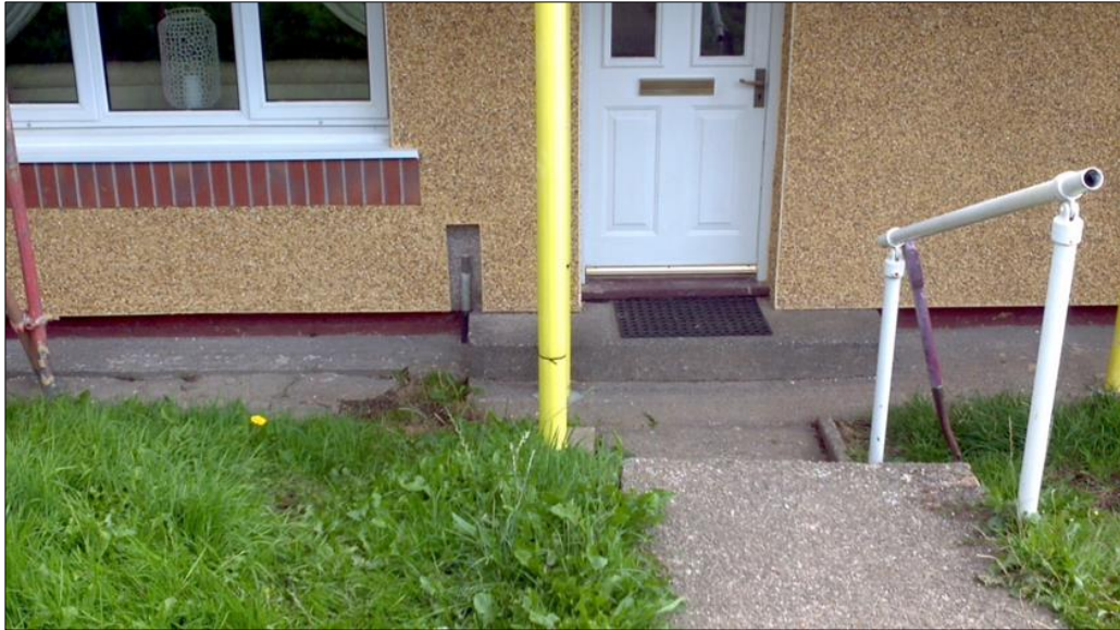
Figure 30: Photograph showing vulnerability of EWI to moisture cause by lack of offset over doorstep
