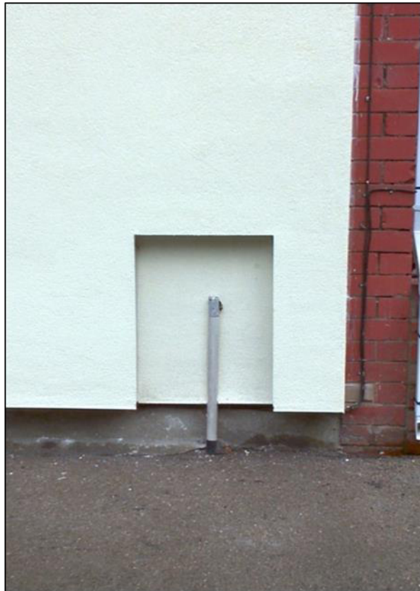
Figure 23: Photograph showing uneven spacing around gas supply pipe
