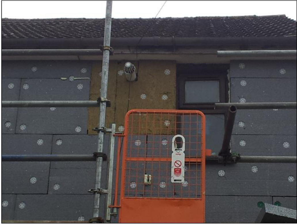
Figure 42: Photograph showing boiler flue projecting through EWI system
