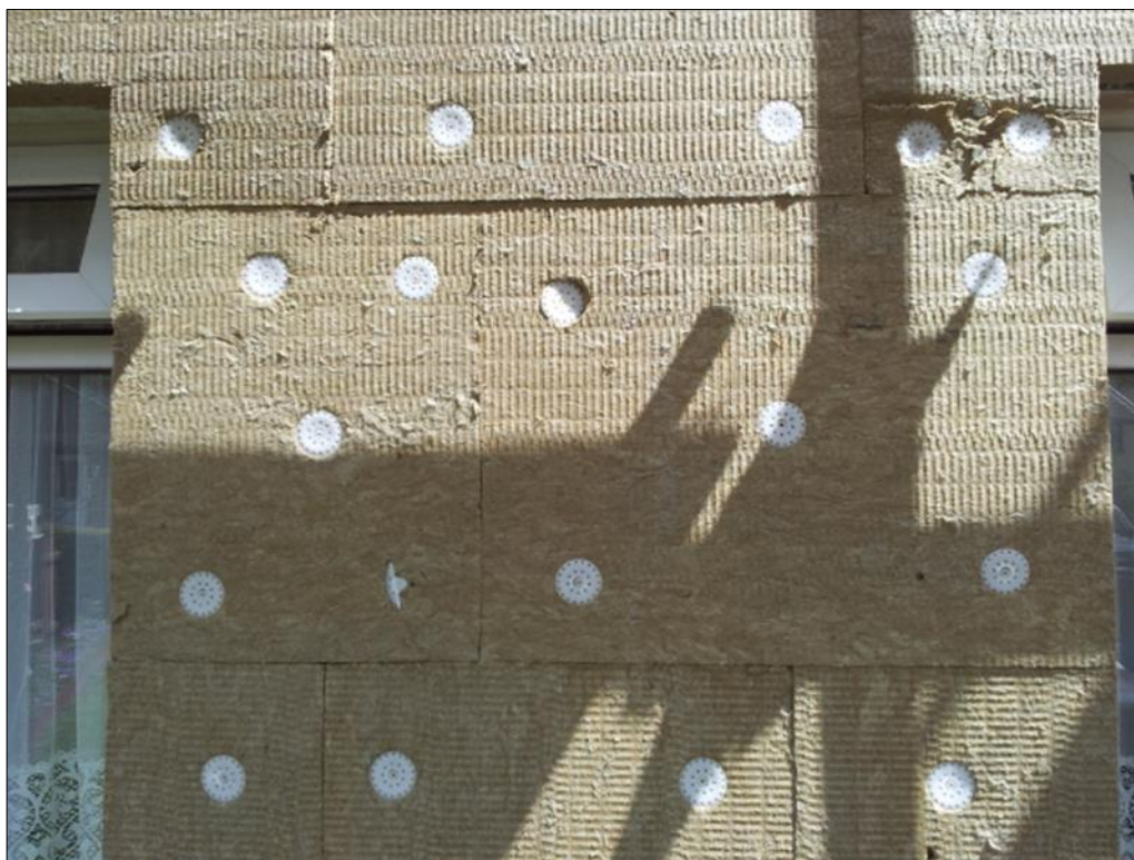
Figure 41: Photograph showing multiple instances of improper pinning
