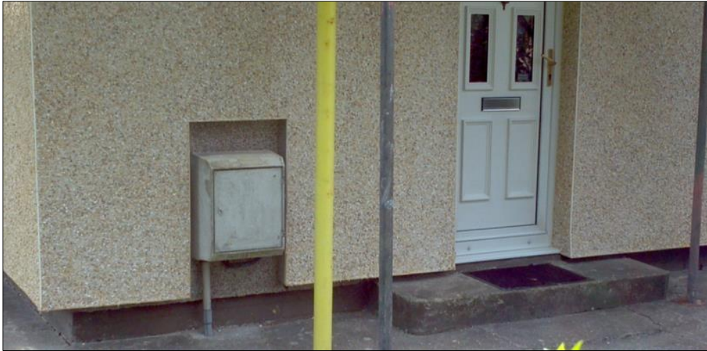
Figure 28: Photograph showing appropriate practice offsetting EWI over doorstep to protect from moisture
