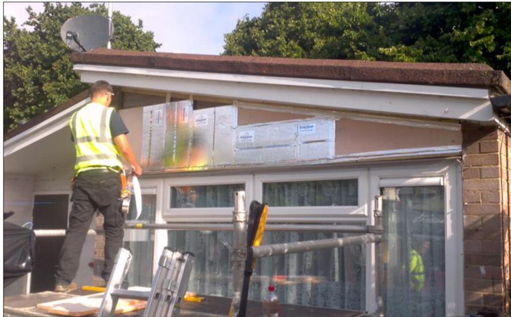
Figure 40: Photograph showing limitations of standardised dimensions of vacuum insulation panels
