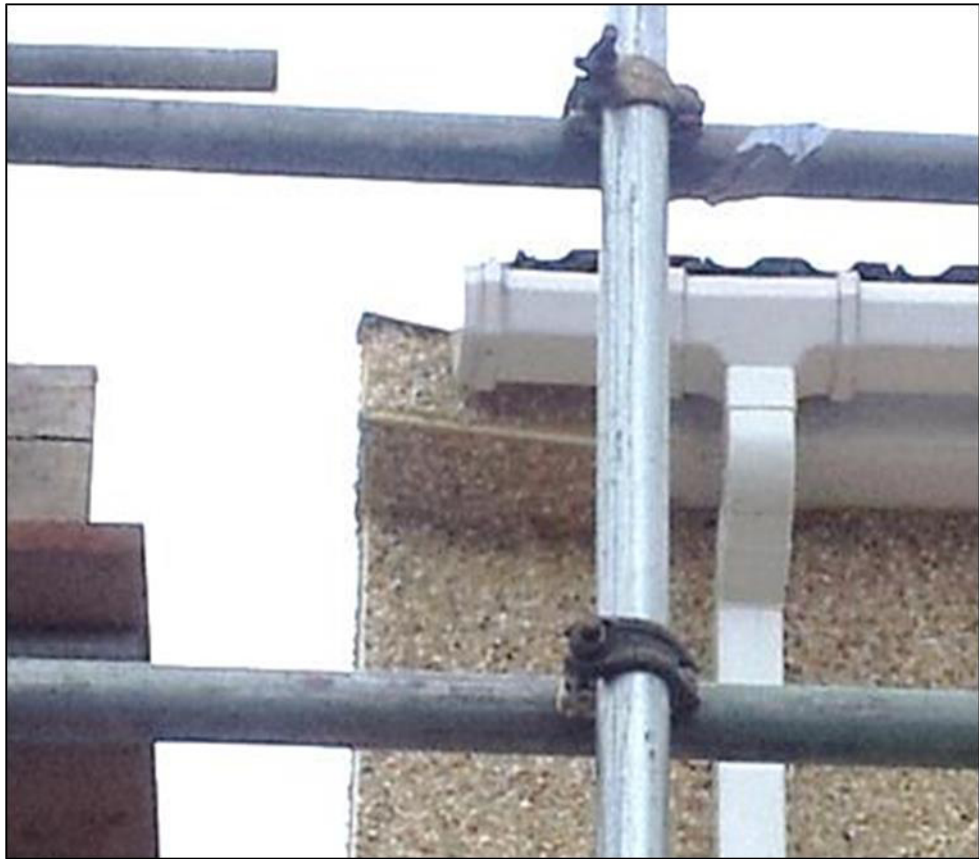
Figure 25: Photograph showing improperly installed verge cap
