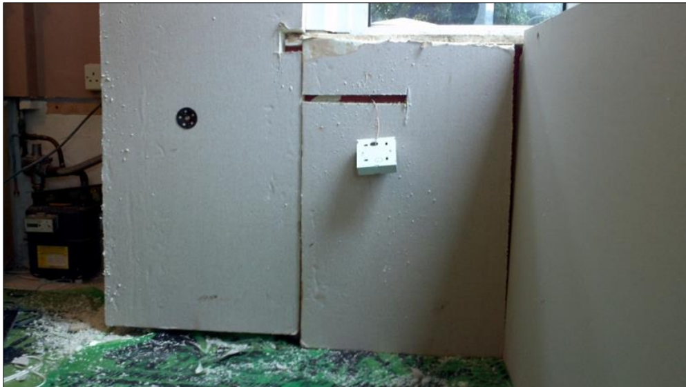
Figure 34: Photograph showing IWI installation with multiple gaps
