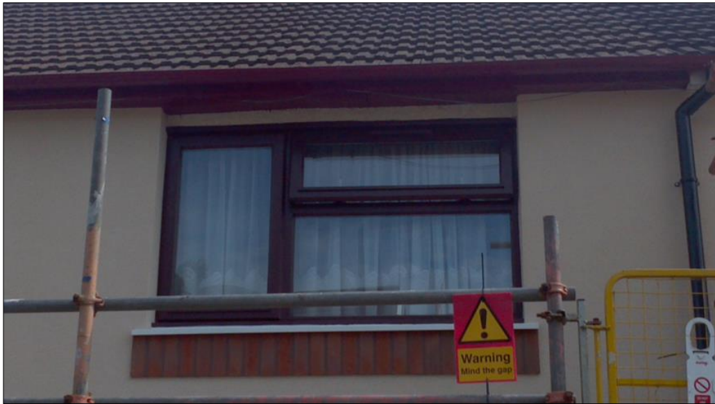
Figure 52: Photograph showing uninsulated window header
