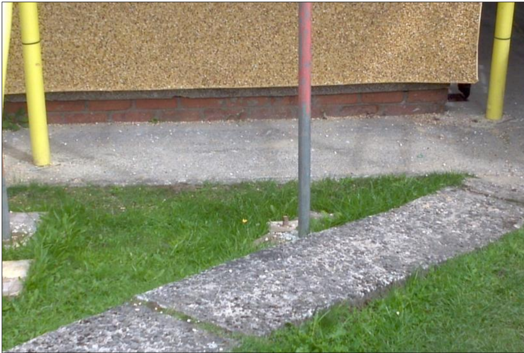
Figure 49: Photograph showing EWI system not covering wall-floor junction
