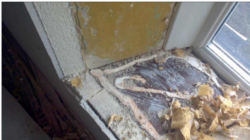
Figure 53: Photograph showing window reveal in IWI system. Note minimal clearance around existing window and lack of insulation installed in reveal.
