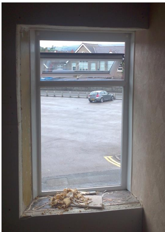
Figure 61: Photograph showing uninsulated window reveal and existing window with narrow clearance and abutting party wall
