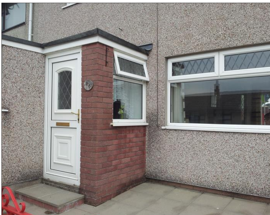
Figure 58: Photograph showing problematic window and door position, seen prior to EWI installation
