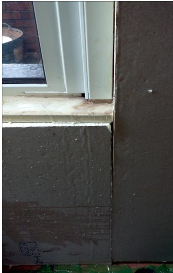
Figure 37: Photograph showing gap and unevenness between two IWI boards, joint between boards at window edge and moisture resulting from poor handling on site
