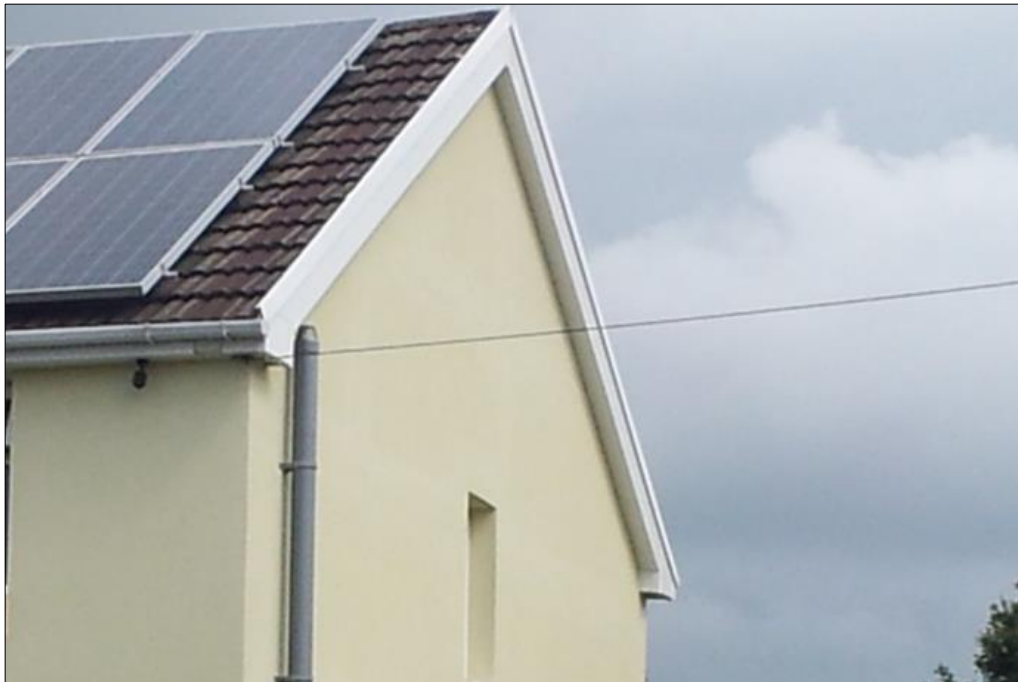
Figure 43: Photograph showing improper installation of soil and vent pipe
