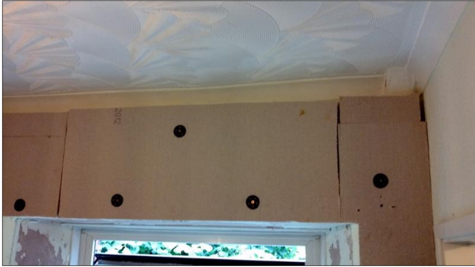
Figure 36: Photograph showing numerous faults in IWI installation
