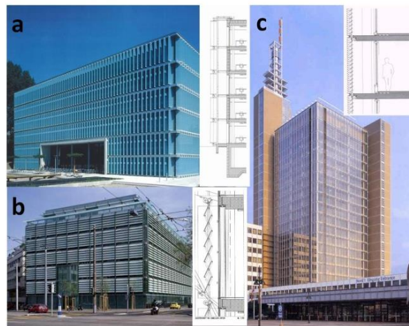
Fig.4 Adjustable external blind systems in (a) EMPA, (b) Ta-Media offices in Zurich, and a mid-pane system in (c) Hannover EXPO HQ.
