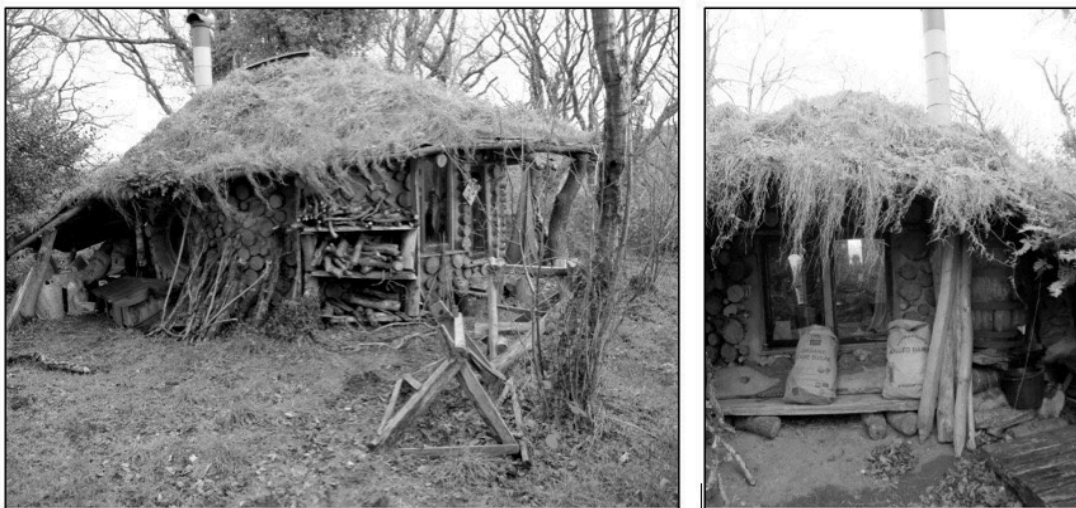
Fig. 4.1 One of several roundhouses on the site, with overhanging eaves used for storage Source: the author
