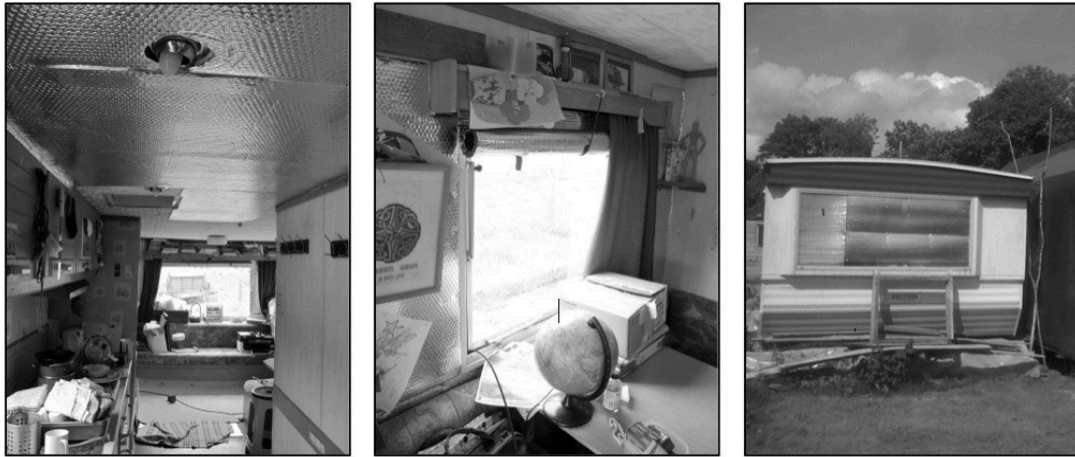
Fig. 6.37 Ad hoc measures to insulate the caravan at UI | Source: the author
