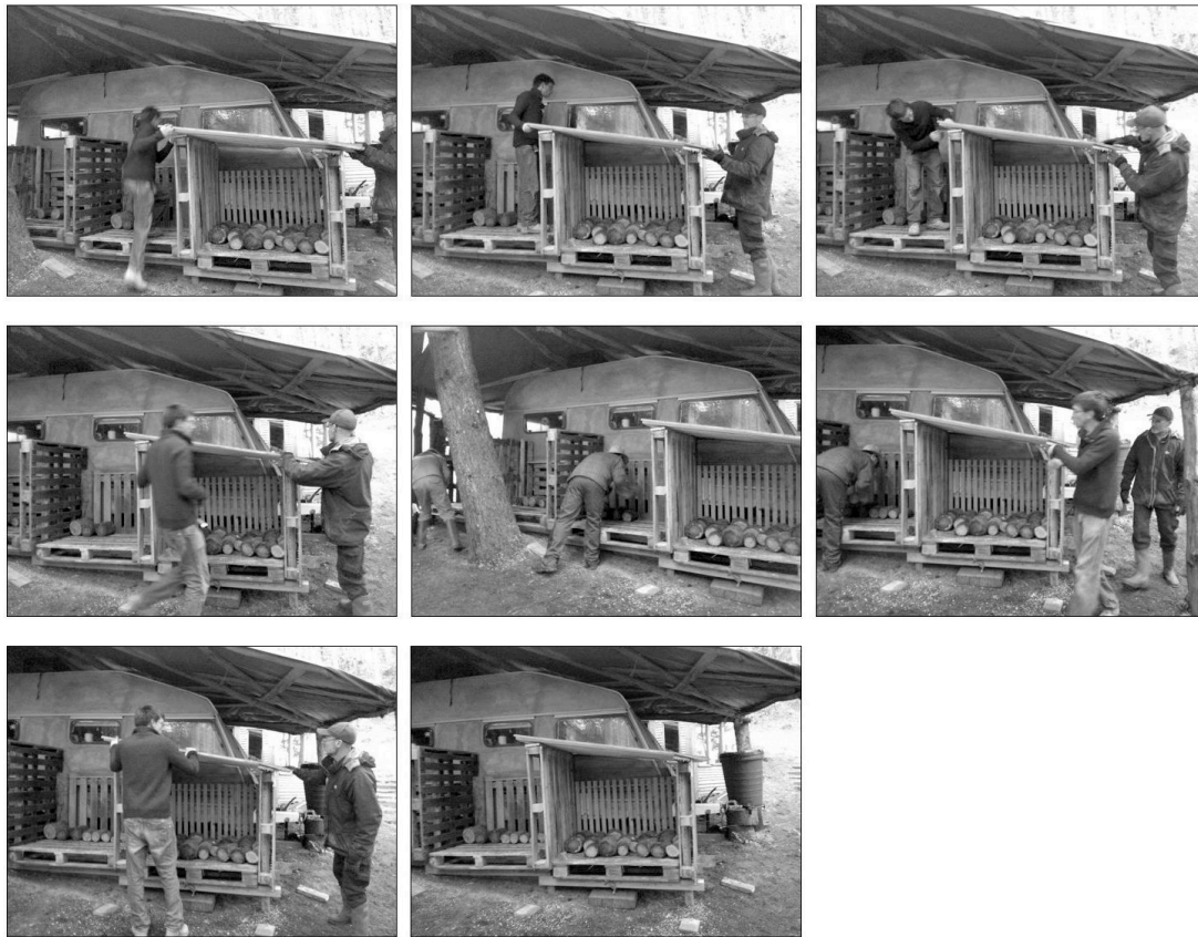
Fig. 6.30 Putting the roof onto the logstore: time sequence 1 Source: anon
