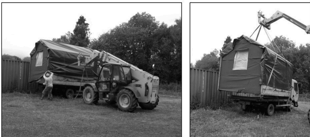
Fig. 6.58 The pod being moved to the new location at BQ | Source: the author
