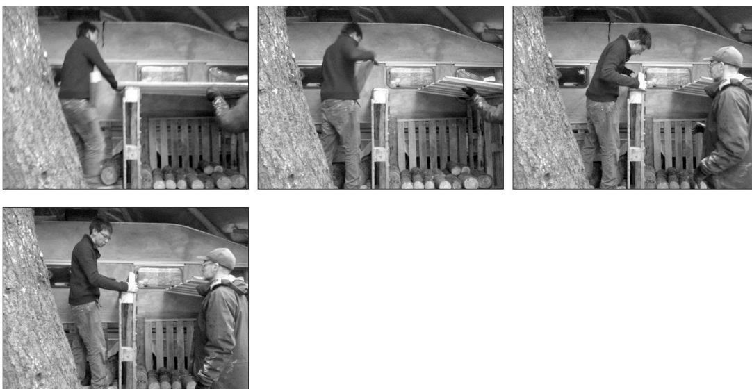
Fig. 6.31 Putting the roof onto the log store: time sequence 2 Source: anon
