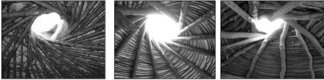
Fig. 4.12 Three roundhouse roofs showing the reciprocal frame and central skylight (the left one is from CN) | Source: the author
