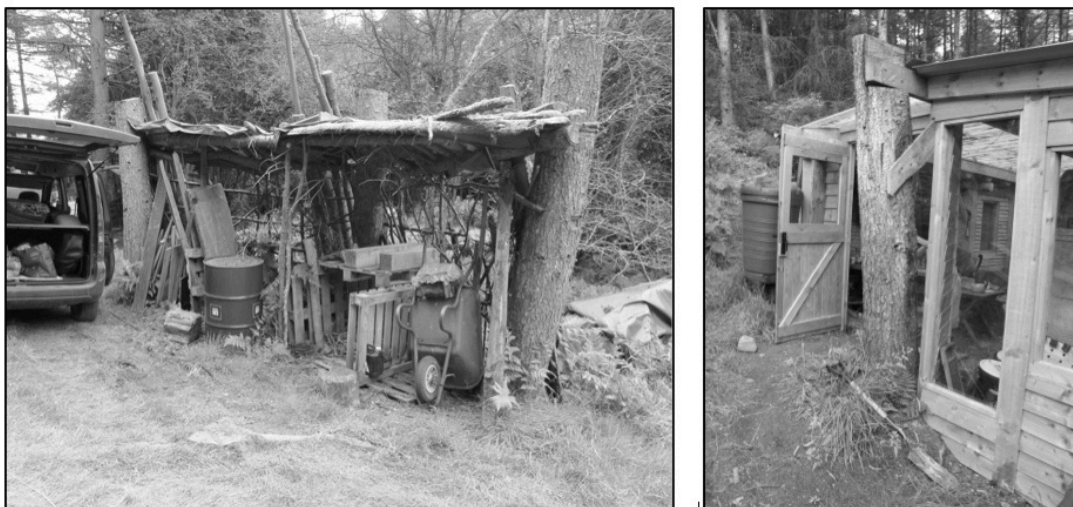
Fig. 6.29 Tree trunks left in situ, acting as columns to support the roofs to the enclosure over the caravan and to a materials store | Source: the author
