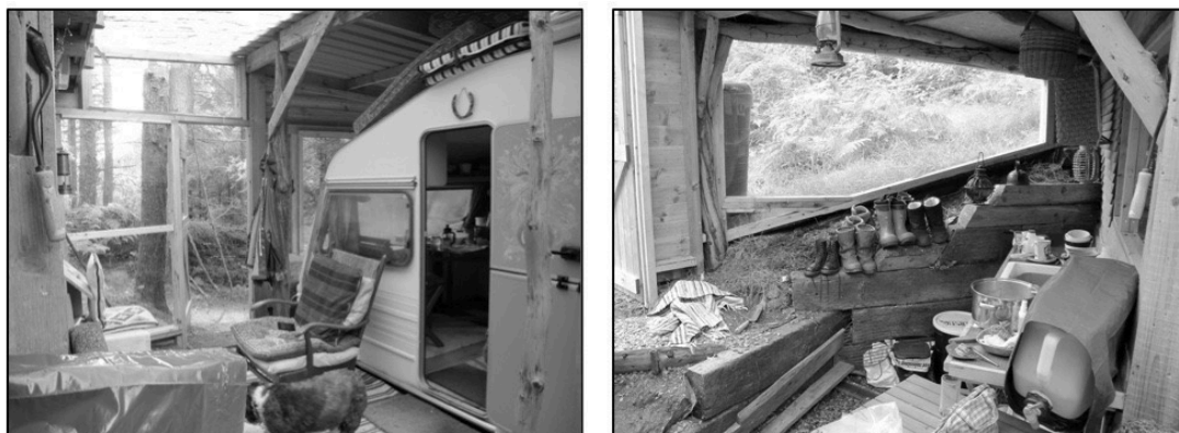
Fig. 6.26 Internal views of the covered area between the caravan and the cabin | Source: the author
