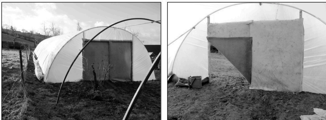
Fig 6.11 Carpets used as ad hoc doors at both ends of the polytunnel | Source: the author
