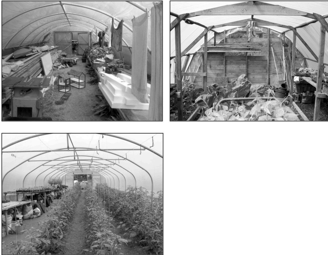
Fig. 4.17 Interiors of three polytunnels from the case studies: HB (top left); OD (top right); and GX (bottom left) | Source: the author
