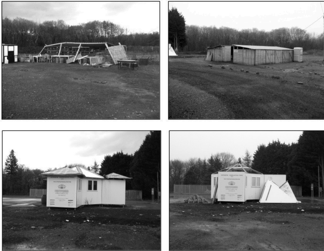
Fig. 6.61 Collapsed poultry auction enclosure, 21/11/2013 (top left); and enclosure rebuilt to revised design, 03/04/2014 (top right); View of modular pod: 21/11/2013 (bottom left); and similar view, 03/04/2014 (bottom right) | Source: the author
