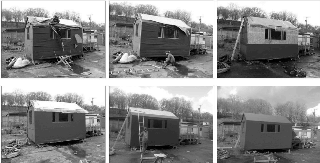
Fig. 6.52 Time sequence showing the process of cladding the pod in vinyl, 24/02/2014 to 27/02/2014 Source: the author
