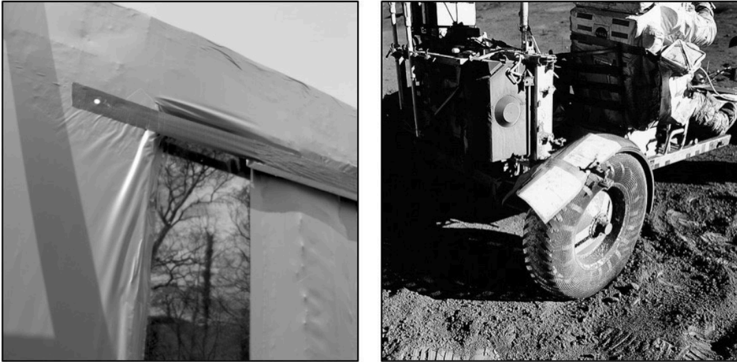
Fig. 7.18 Duct tape used on the pod to form an ad hoc drip detail (left); and duct tape used on the moon during an Apollo landing (right)
