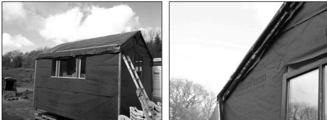
Fig. 6.43 Black polythene being used as a roof finish | Source: the author
