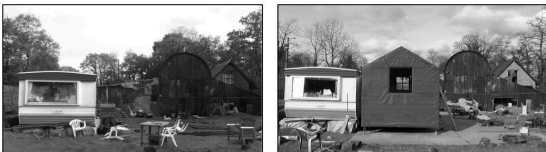
Fig. 6.49 View of UI, looking back at caravan, barn and house: in 2012 (left); and in 2013 during construction of the pod (right) | Source: the author
