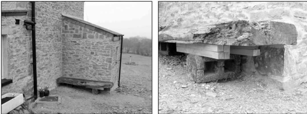
Fig. 6.15 Ad hoc bench at HM resting on concrete blocks and 2x2 timbers originally intended for polytunnel doors. | Source: the author
