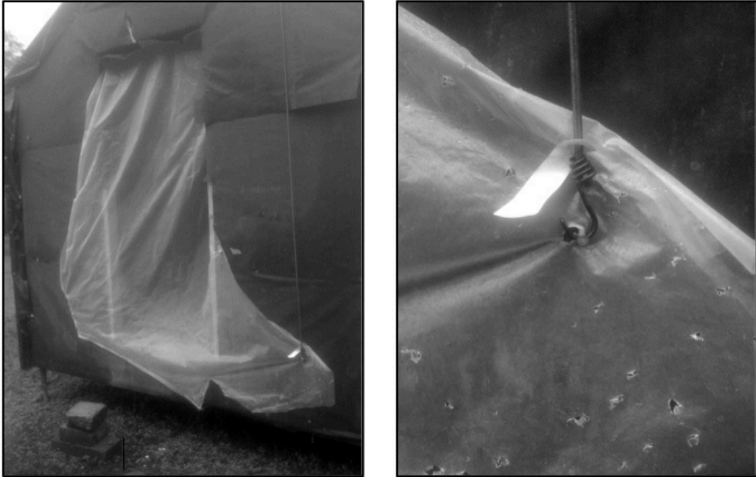
Fig. 6.60 Method used to keep the polythene 'door' in place to the pod at BQ (photograph to the right is a detail showing how a bungee rope was recruited into the task) | Source: the author
