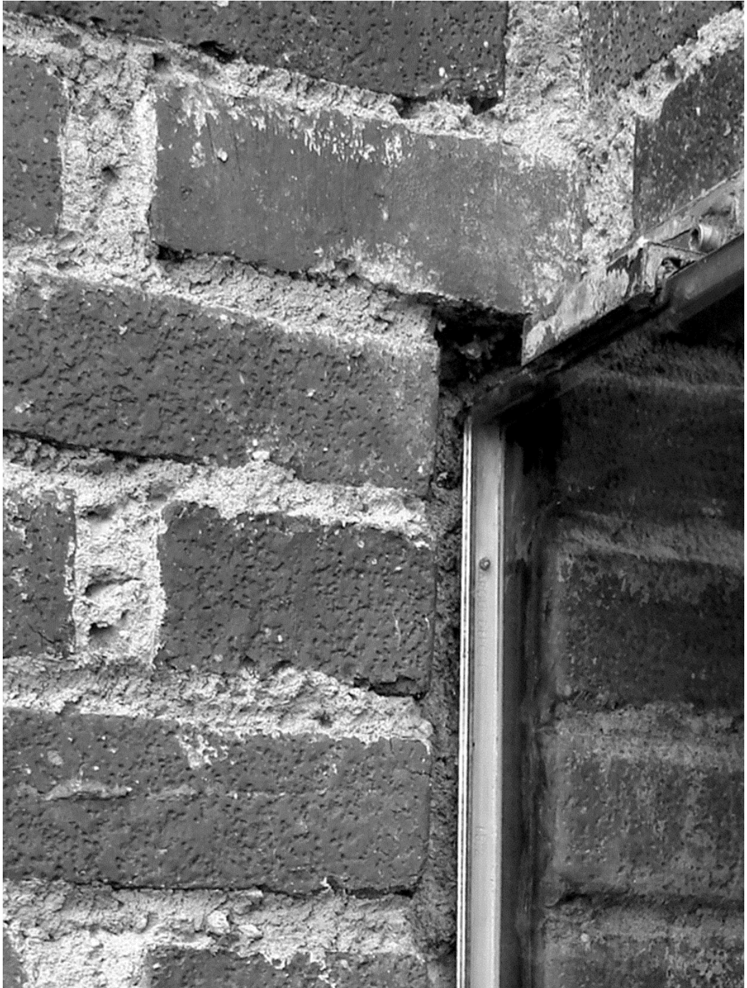
Fig. 1.1 - Mortar joints at St Peter's, Klippan.
