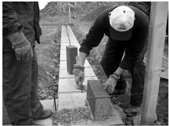
Fig. 2.23 - Concrete block foundation wall of the north addition, Wheelingstone, 2004.
