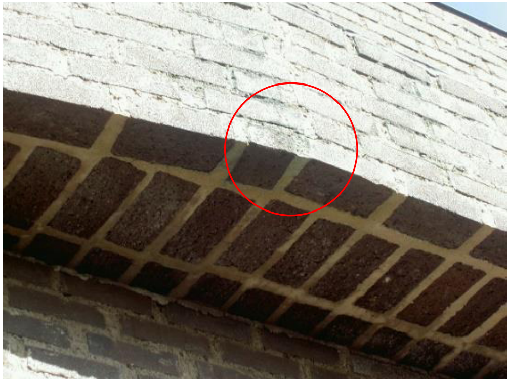
Fig. 3.15 - Deviation from a stringently applied rule: a cut brick, close-up, observed and photographed by Simon Unwin.
