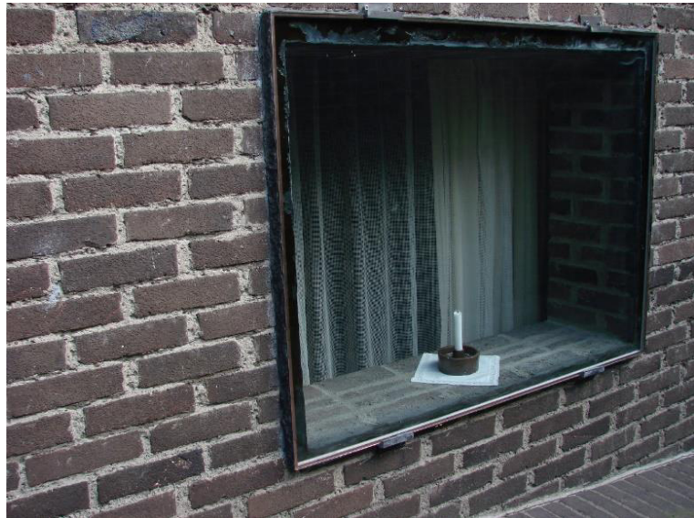
Fig. 3.9 - Window detail at St Peter's.
