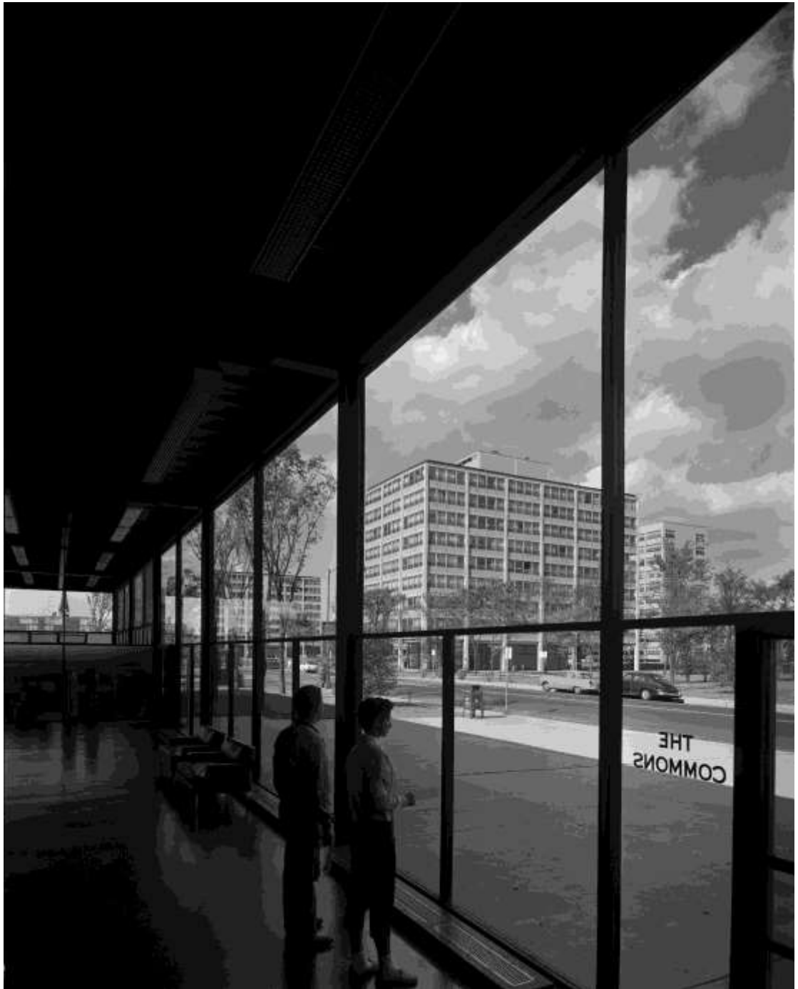
Fig. 9.11 - Commons interior, showing the full height steel muntins referenced by Friedman's letter highlighting concerns raised by FAS's structural engineers [This image is titled 'apartment / dormitory buildings: Chicago, (Ill), referencing the Graduate Halls which are visible externally], Hedrich-Blessing (photographer) © Chicago History Museum: HB - 18783-C.
