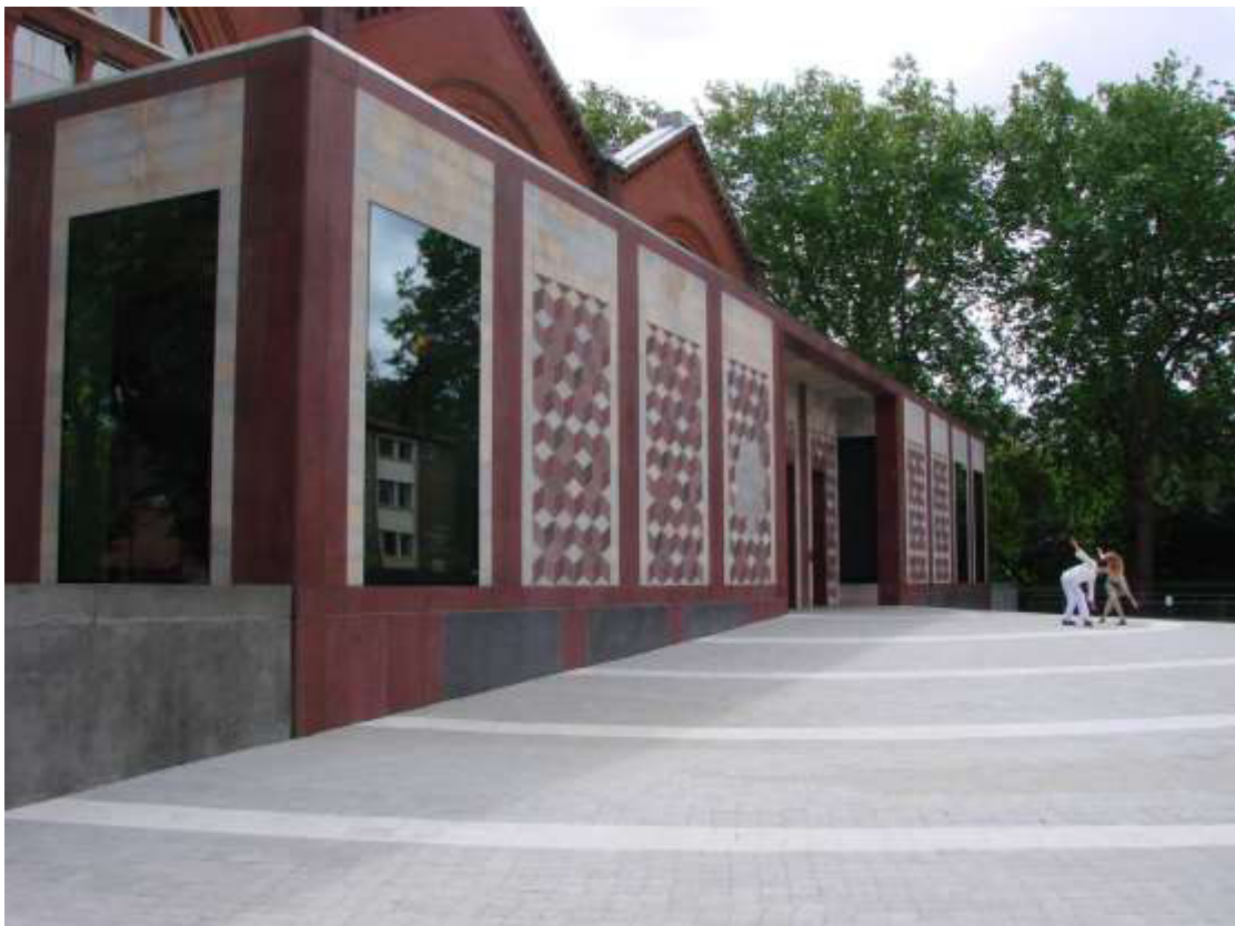
Fig. 8.31 - Constructed west façade, Museum of Childhood, Caruso St John Architects.
