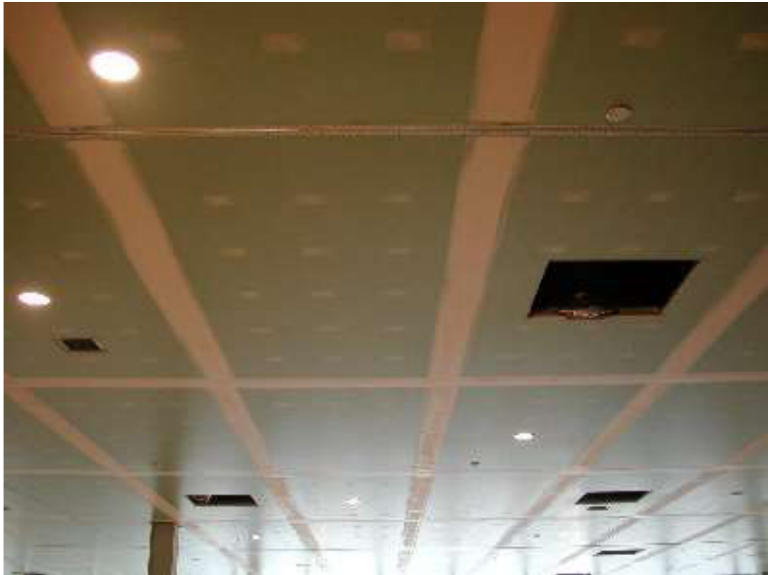
Fig. 10.29 - Photos 03/05/03 #1/2 Image sent by Mark Schendel to highlight 'the differential drying of the sealer'
