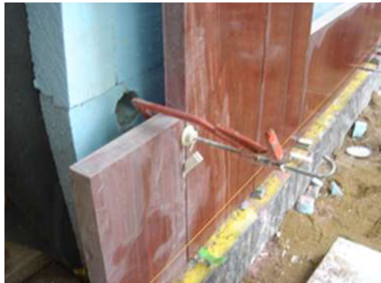
Fig. 8.22 - Construction of stone cladding underway. 176_120906_03. Caruso St John Architects..
