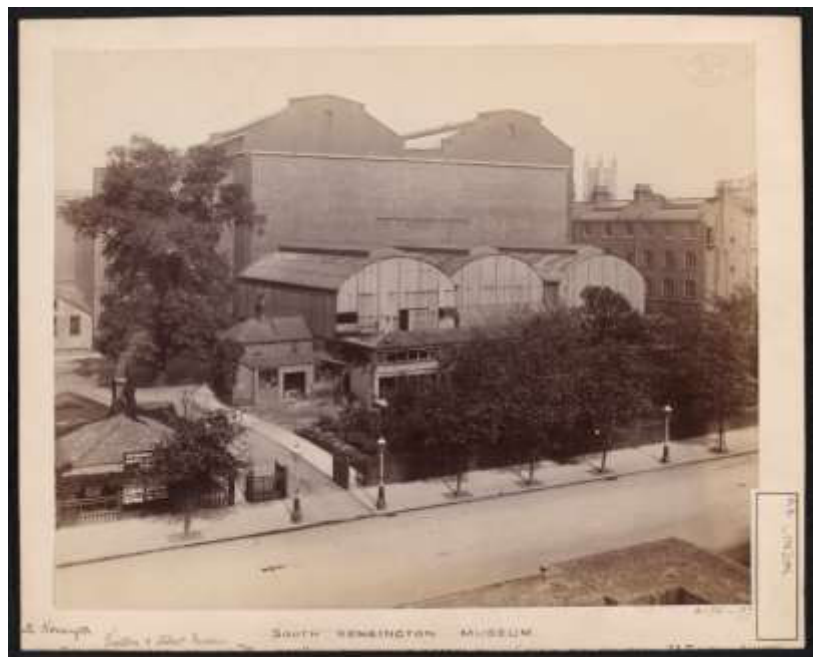
Fig. 7.16 - South Kensington Museum, remains of the 'Brompton Boilers', south of the Cast Courts, under demolition with Secretariat block on left, the Cast Courts in background and tower of Holy Trinity Church in distance. 1897. Commissioned by Department of Science and Art of the Committee of Council on Education. © Victoria and Albert Museum: No.PH.4176-1897.
