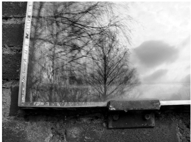
Fig. 3.11- Window detail at St Peter's.
