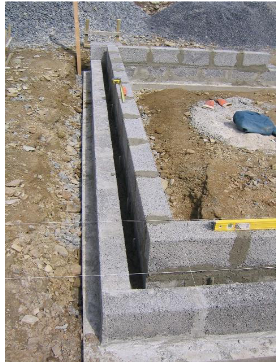
Fig. 2.24 - Concrete block foundation wall of the north addition, Wheelingstone, 2004.
