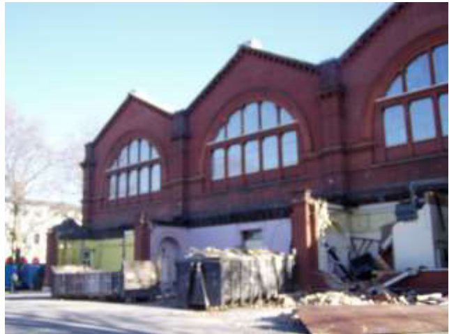
Fig. 8.19 - Demolition of Wild's colonnade complete. 176_sitephoto_090206_03. Caruso St John Architects.
