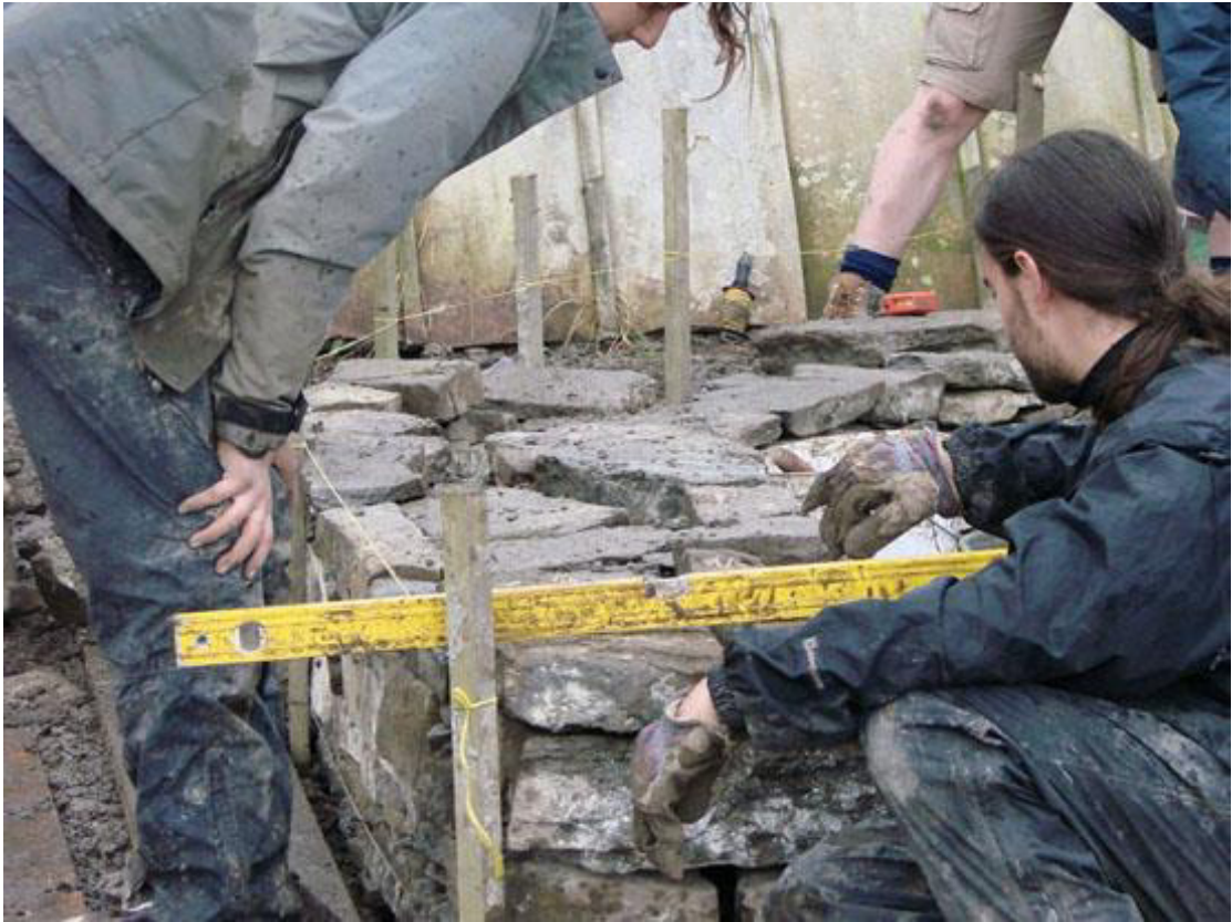
Fig. 4. 1 - Spirit level on a flagstone wall. Welsh School of Architecture undergraduate students Madeline Kinderman and Alex Whitcroft building a 'boat nose' at Westray Heritage Centre, Westray, Orkney Islands, in a 2007 workshop led by Mhairi McVicar.
