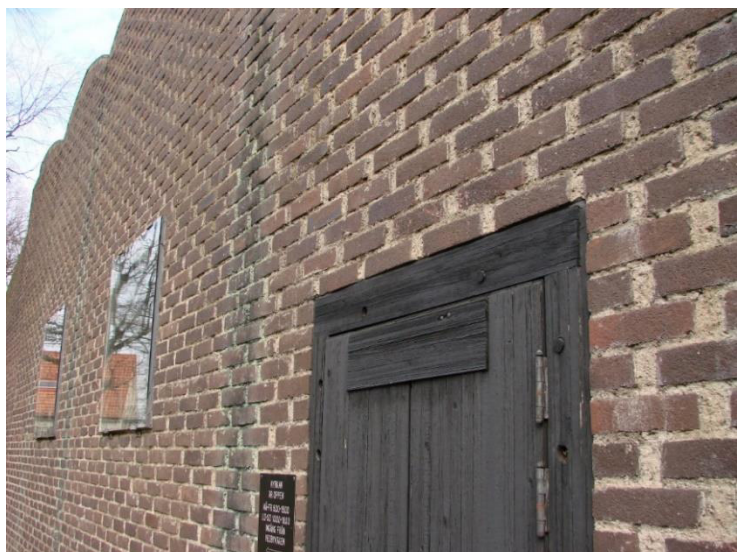
Fig. 3.8 - Mortar joints at St Peter's, exterior.
