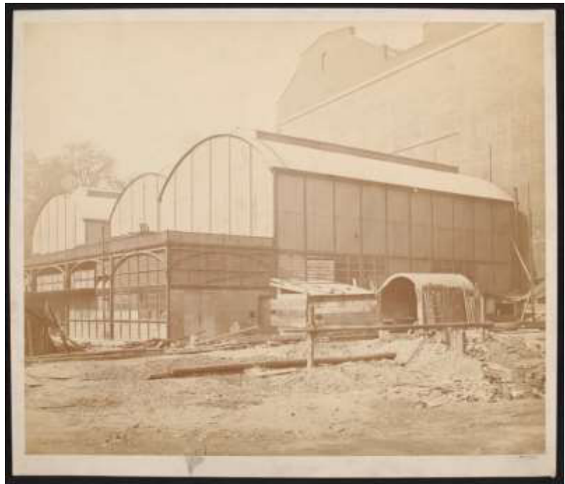
Fig. 7.15 - External view of 'Brompton Boilers' at South Kensington before removal to Bethnal Green, showing Cast Courts in background. 1872. Isabel Agnes Cowper photographer. Commissioned by Department of Science and Art of the Committee of Council on Education. © Victoria and Albert Museum: No. 72:431.
