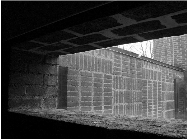
Fig. 3.10 – Window detail at St Peter's.
