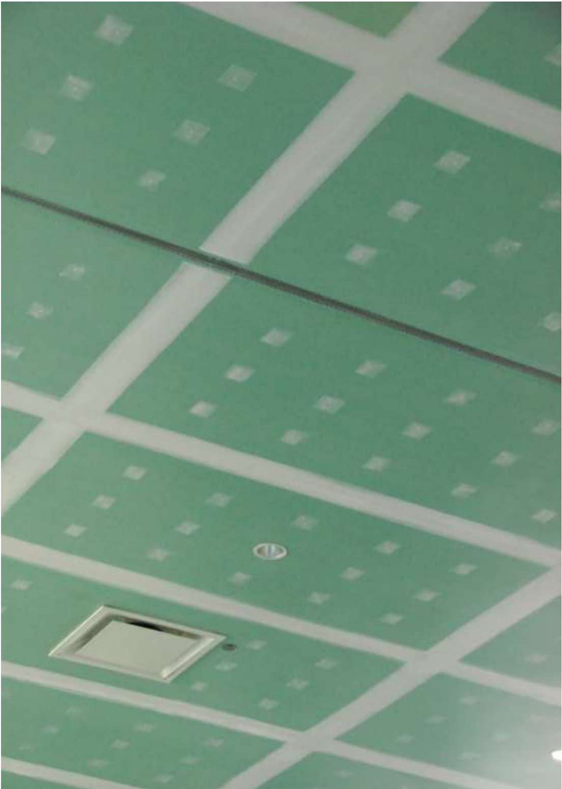
Fig. 10.1 - 'IIT' Green Board ceiling, McCormick Tribune Campus Centre, photographed 2010.
