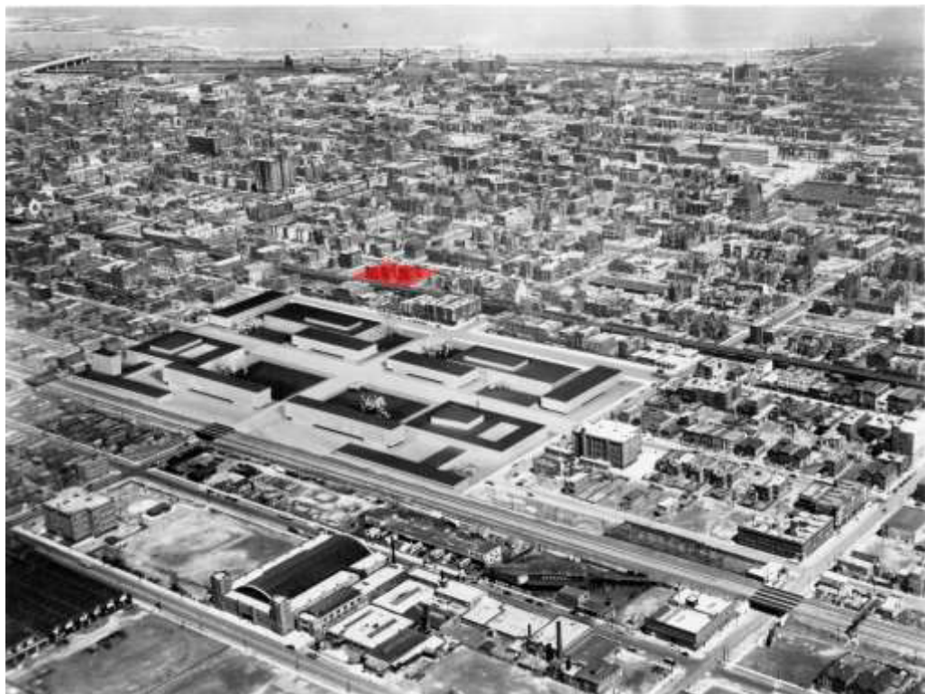
Fig. 9.5 - Campus development aerial view proposed campus, IIT [looking north-east]. Kaufmann & Fabry Co. (photographer) photo No. 962 (Ca 1941) Chicago 41-2022-2. University Archives and Special Collections, Illinois Institute of Technology, Galvin Library. 1998.277 IIT Aerial Photos Binder 1 1940-1951 (1941) Image #2.1. The site of the Commons is shown in red (added by author).
