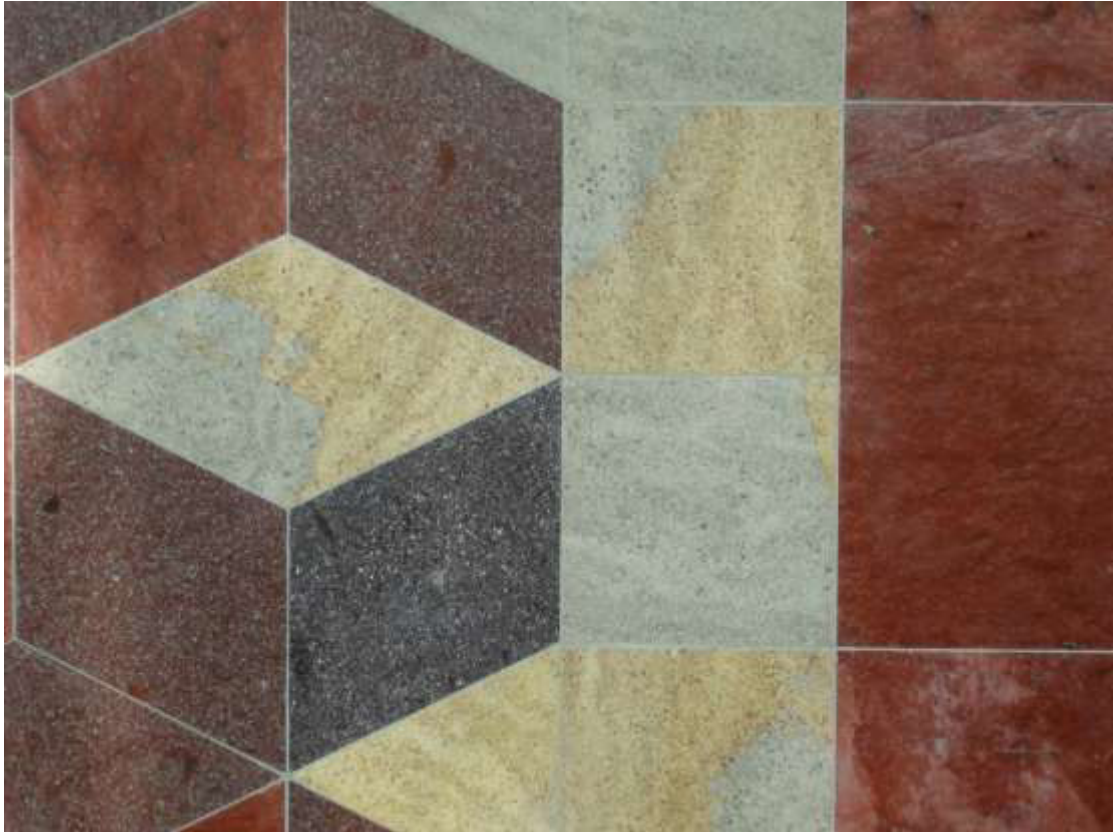
Fig. 8.32 - Detail of constructed west façade of the Museum of Childhood entrance addition. Site Photos / Stone 14.7.05 /DSC00230.jpg, Caruso St John Architects.
