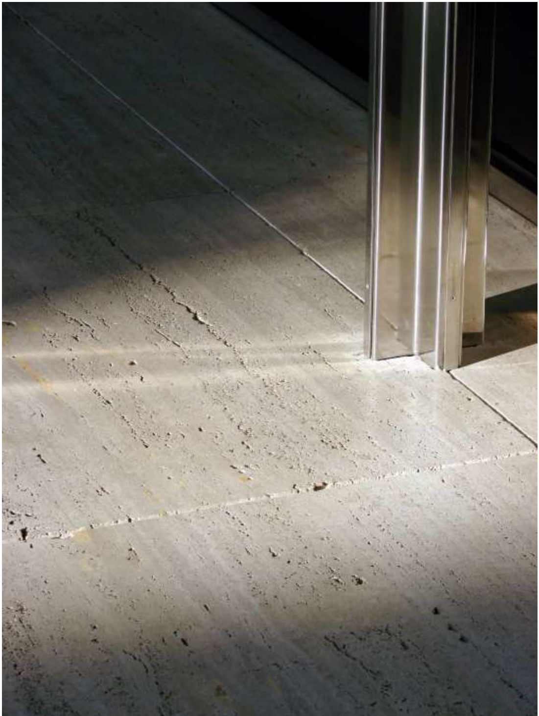
Fig. 9.3 - Barcelona Pavilion reconstructed column, photographed 2008.
