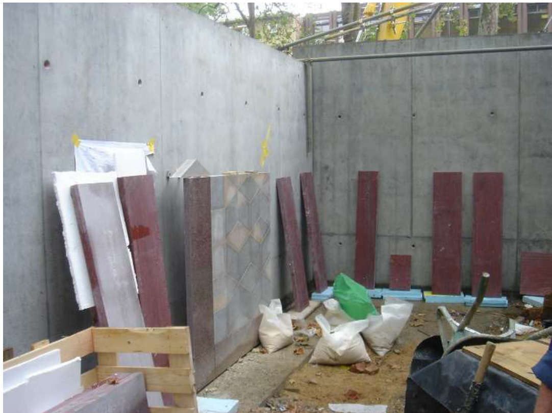
Fig. 8.20 - Façade panel sample constructed on site. 176_120906_07. Caruso St John Architects
