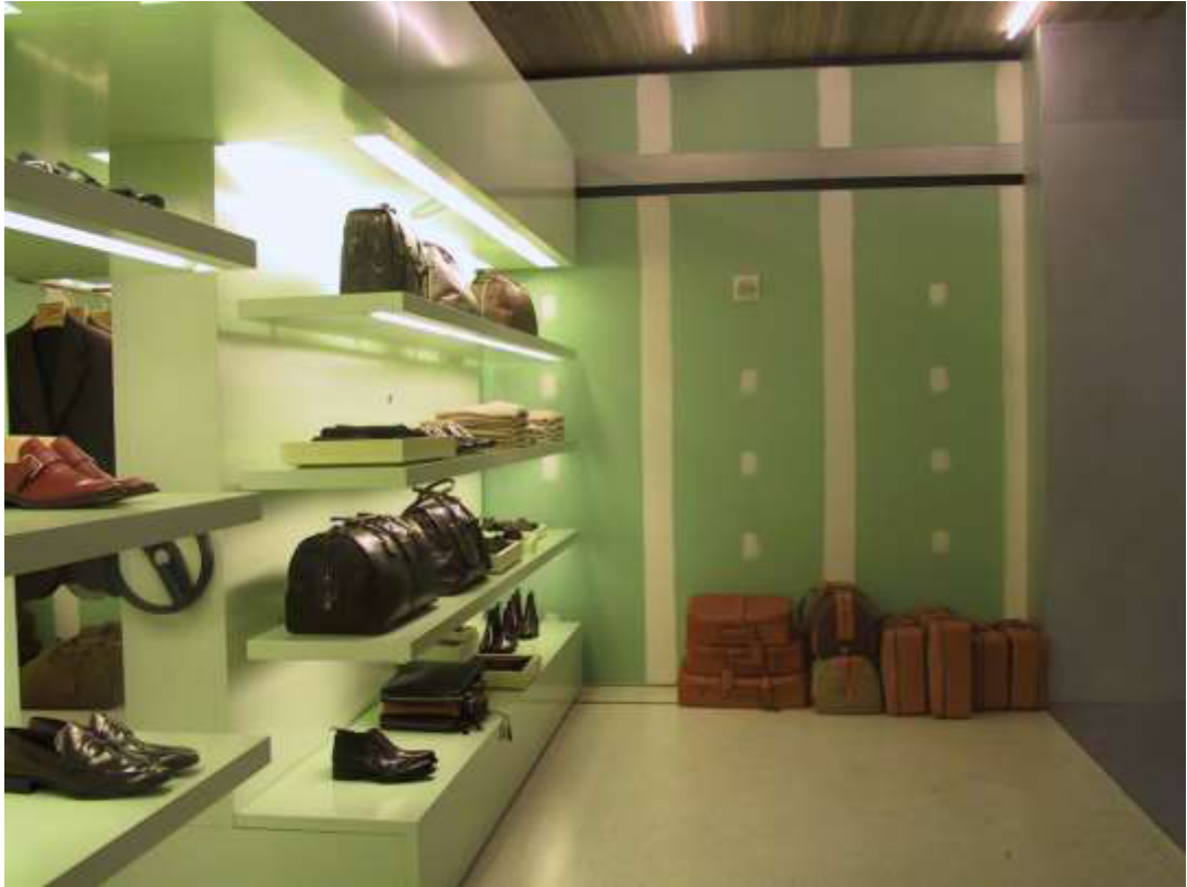
Fig. 10.15 - Exposed Greenboard wall at Prada New York. Forwarded to Greg Grunloh by OMA NY on 1 January 2002.
