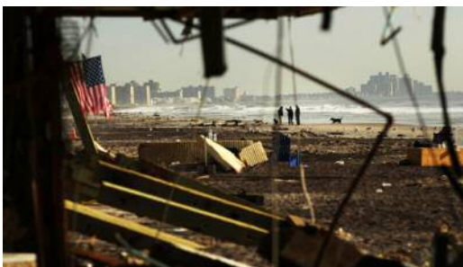
The Morning After – Cables Everywhere
