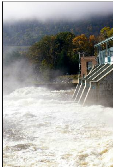
Figure 7: Hydro Energy Generator Facility
