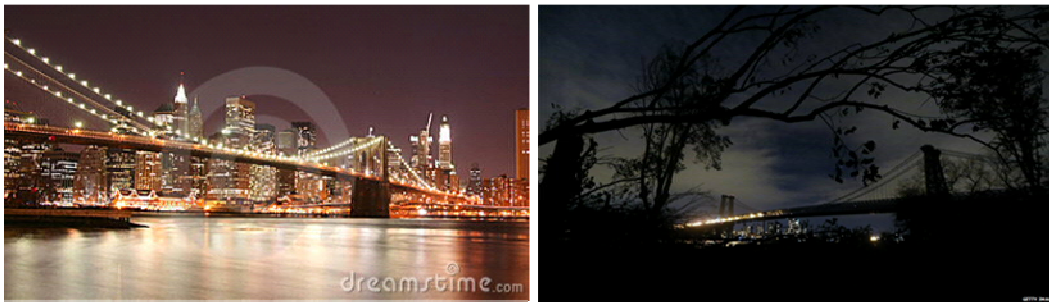
Figure 26: Brooklyn Bridge at Night (left); Power Outage during Hurricane Sandy on the Brooklyn Bridge and Change in Place Perception (right)
