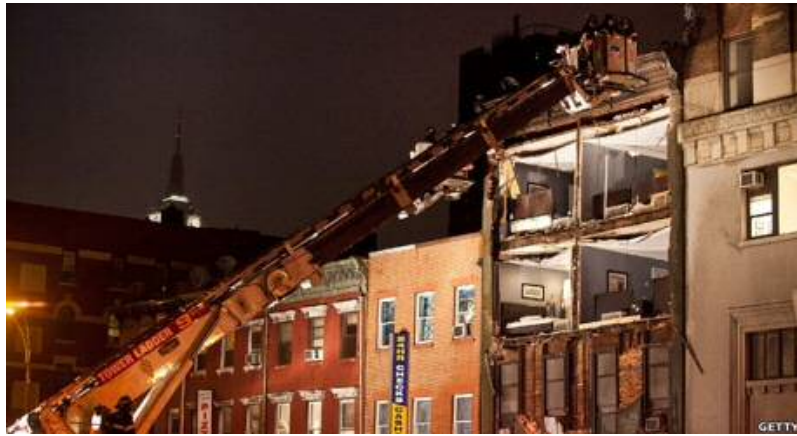
Figure 36: Electricity Cables Displayed in a Ripped House with no Face in Manhattan
