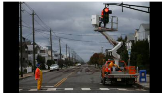
Recovery Efforts – Restorations of Traffic Lights
