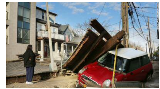
Fallen Power Lines Damaged Property as well as Caused Electricity Loss
