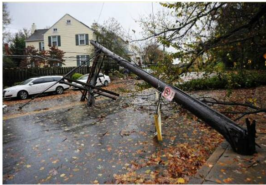
Fallen Energy Pole post-Sandy
