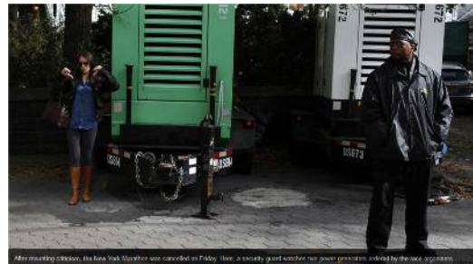
Generators for the Public
