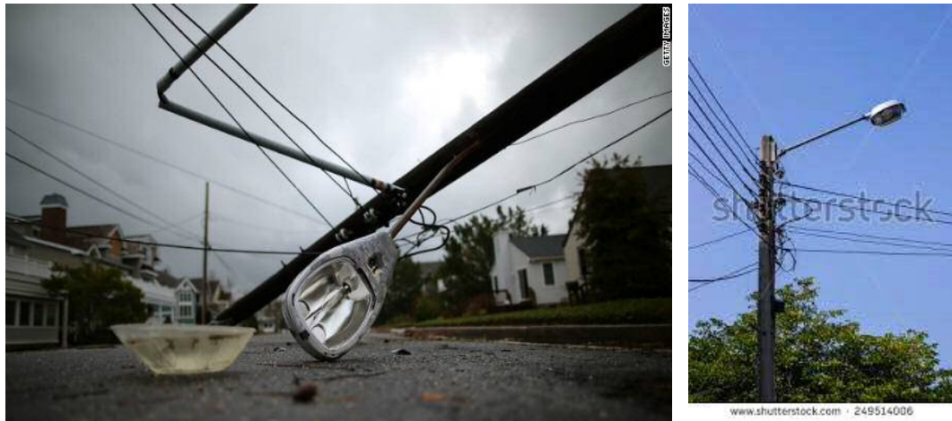
Figure 39: Fallen Power Lines that Lead to Loss of Electricity for Both Private and Public Spaces (left); Power Lines Upright as ‘Norm’ (right)
