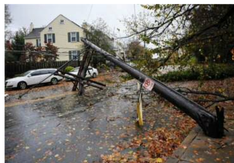
Fallen Electricity Lines
