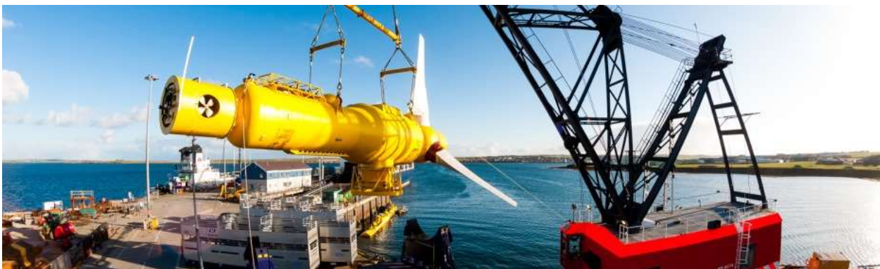
Figure 1.13 Deployment of Alstom Ocean Energy 1 MW device at EMEC (Alstom Ocean Energy, 2013)
