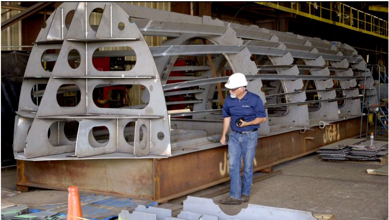
Figure 1.20 Fabrication of Verical Spars by Aecon Atlantic Industrial Inc. (Black Rock Tidal Power, 2016)
