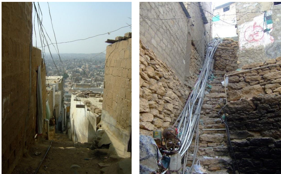
Figures 3: Winding street pattern and illicit water and electricity connections in Chamra Chum, North Nazimabad
